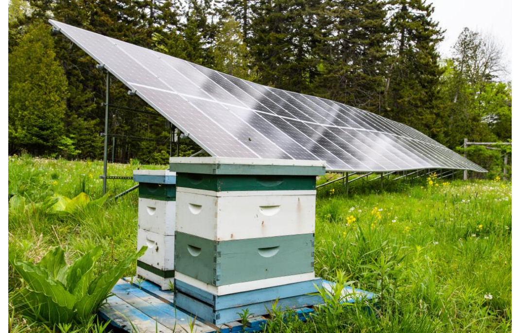
Solar panels at the Islesboro Central School. (Photo by Bryan Bechtold/NREL)
