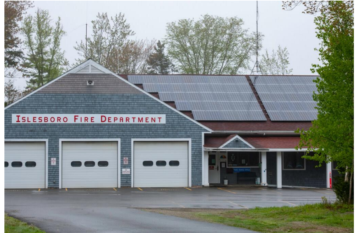
Solar panels on the Islesboro Fire Department. (Photo by Bryan Bechtold/NREL)
