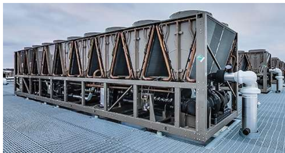
Figure 15: Large Rooftop Chiller Unit for Data Center [20].
