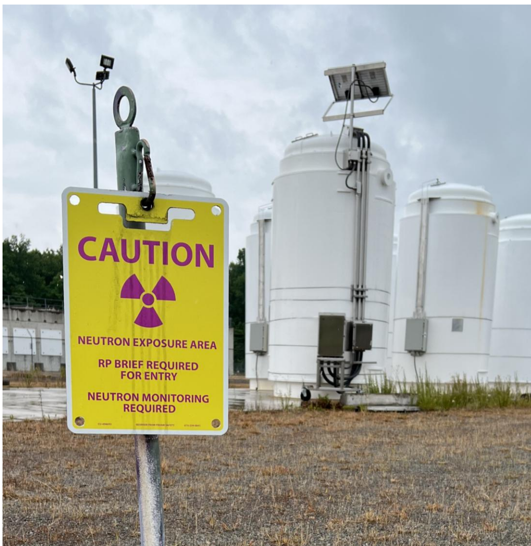
Figure 1-1. TN-32 storage casks at the North Anna Power Station site independent spent fuel storage installation (showing the TN-32B HBURC with solar panel).
