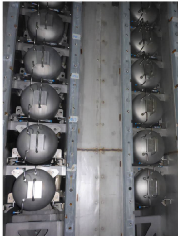
Figure 5-2. Example Delay Tanks from the Australian Nuclear Medicine Active Ventilation System (Hoffman and Brink 2021).
