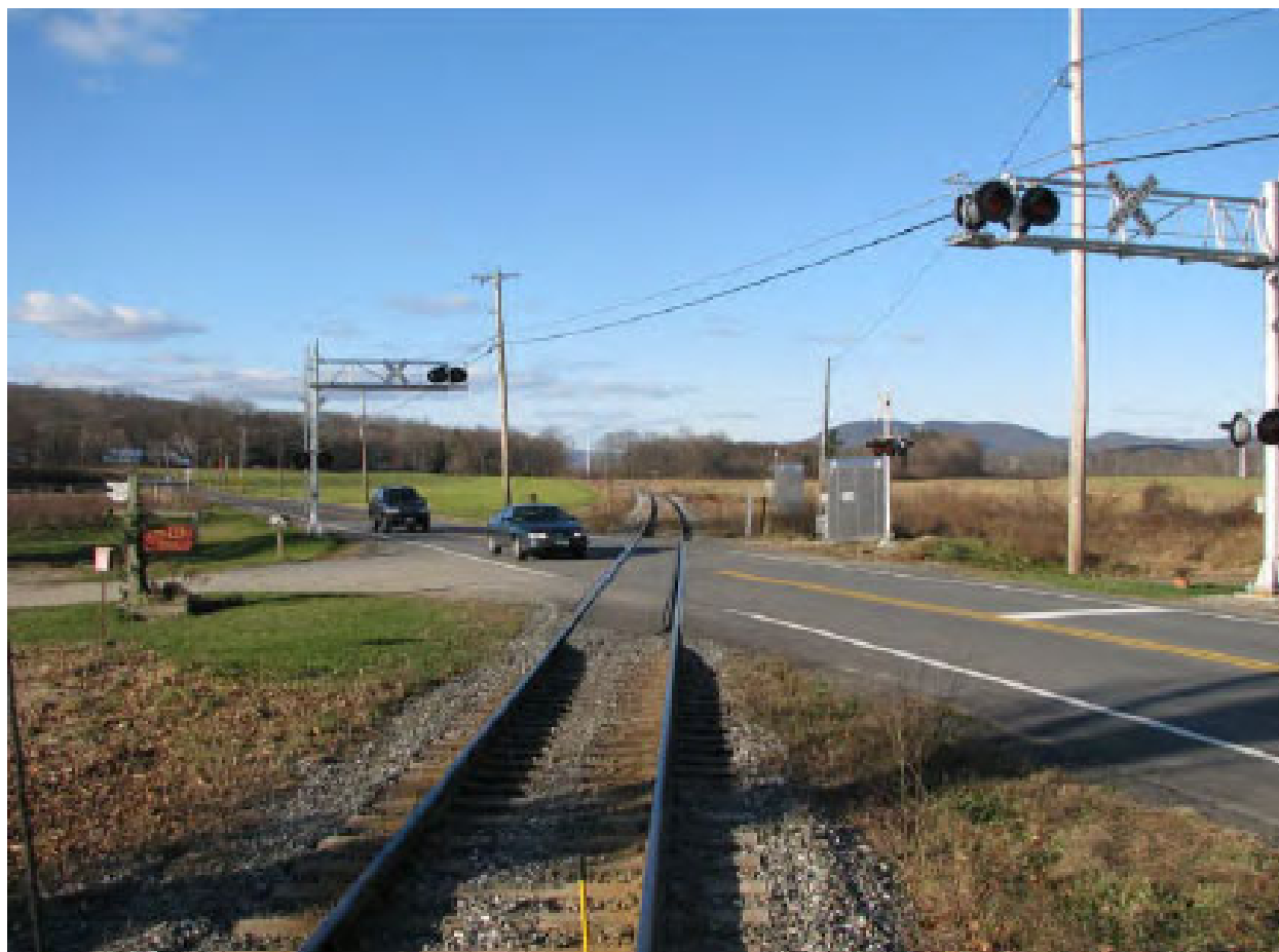
Figure 2-11: State Route 142 Grade Crossing at Milepost 115.97, 2008 [6]
