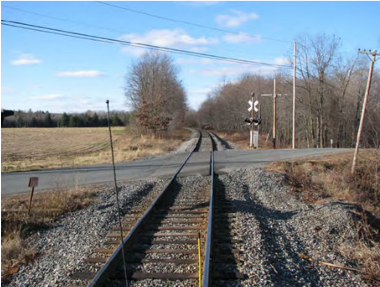
Figure 2-12: Grade Crossing at Milepost 112.68, 2008 [6]
