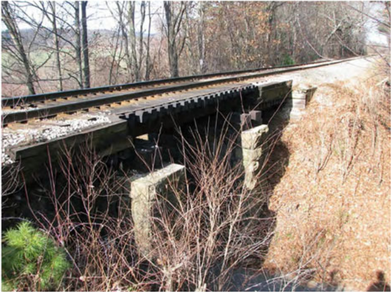
Figure 2-14: Railroad Bridge at Milepost 103.33, 2008 [6]
