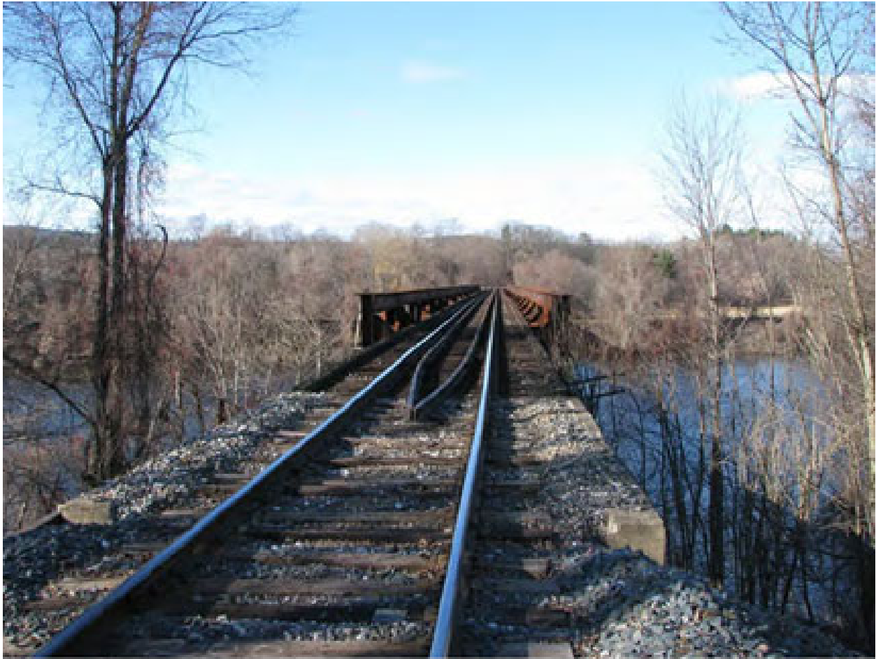
Figure 2-13: Connecticut River Railroad Bridge at Milepost 109.15, 2008 [6]
