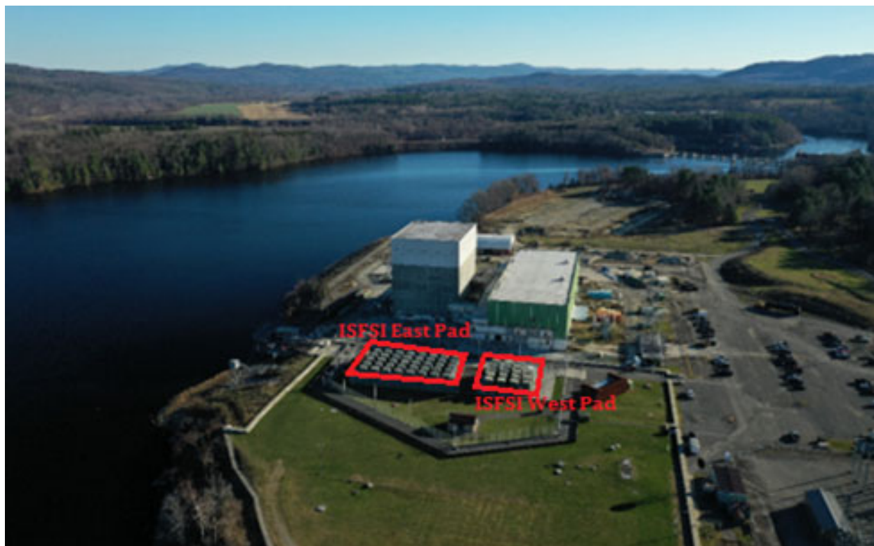
Figure 2-4: VYNPS Elevated Photo Facing South
