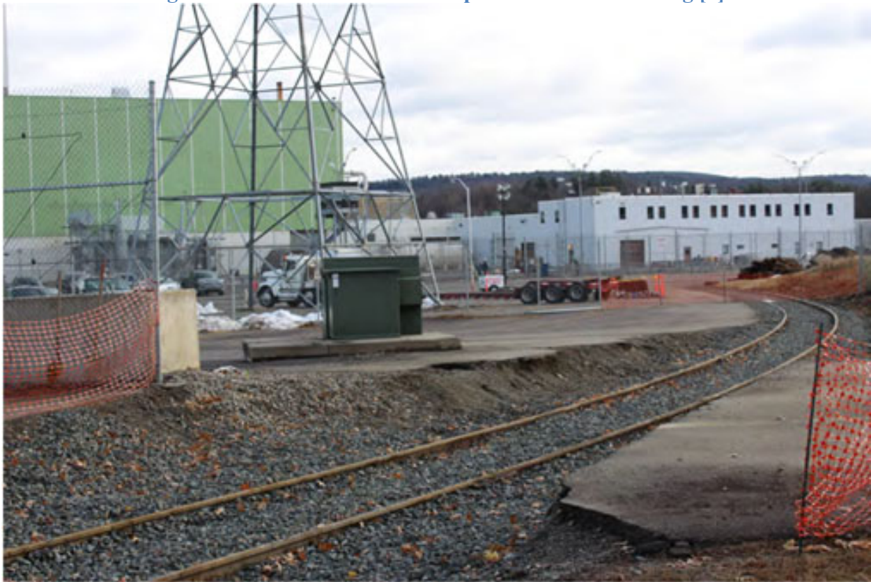
Figure 2-9: VYNPS Onsite Rail Spur to Turbine Building [6]
