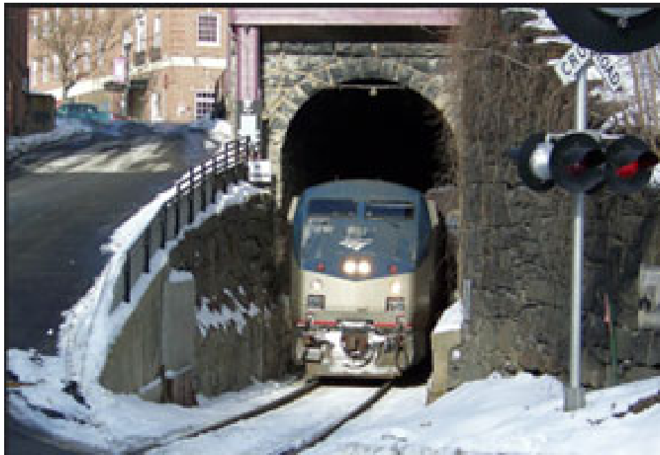
Figure 3-7: Bellows Falls Tunnel with the Vermonter Coming Through [45]
