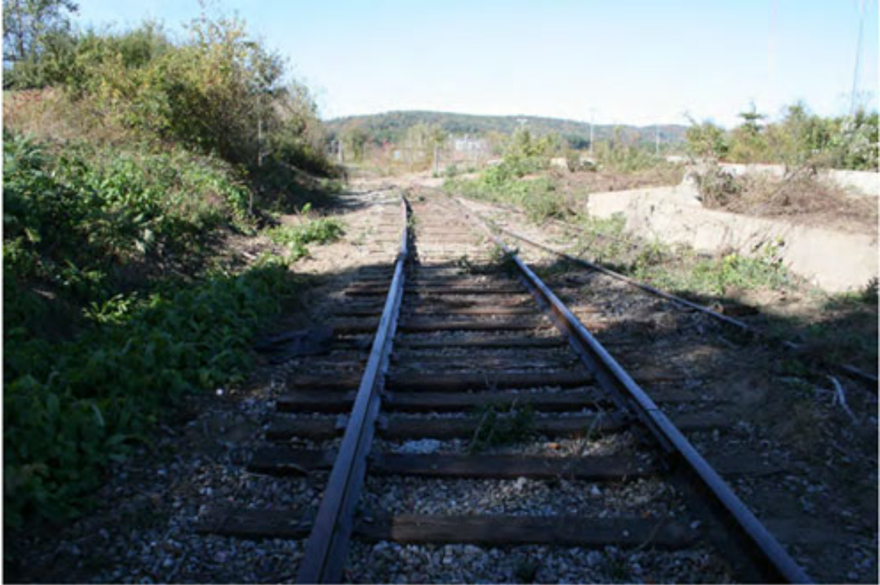
Figure 2-7: Rail Spur Entrance to VYNPS, Right Side Spur goes to Containment Building, Left Side Spur goes to Turbine Building [6]
