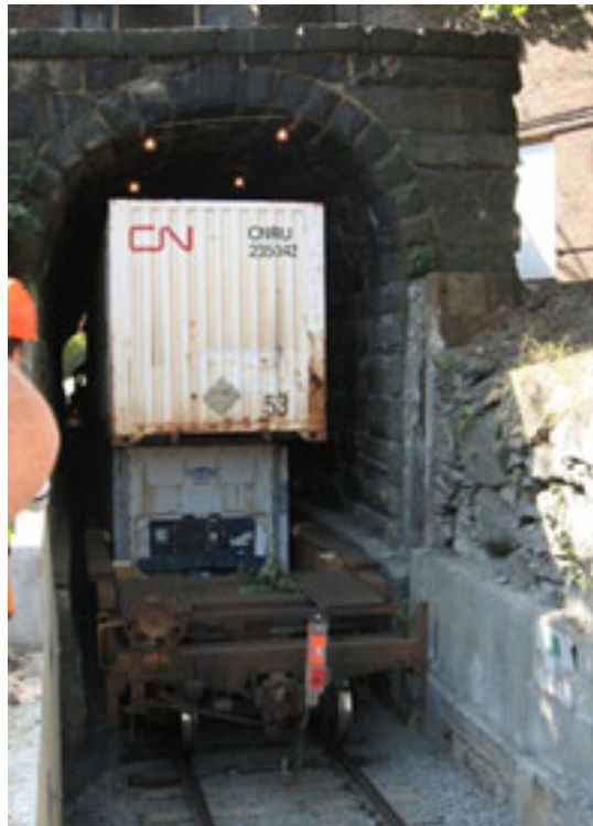
Figure 3-8: Bellows Falls Tunnel with Double Stack Containers Coming Through [47]
