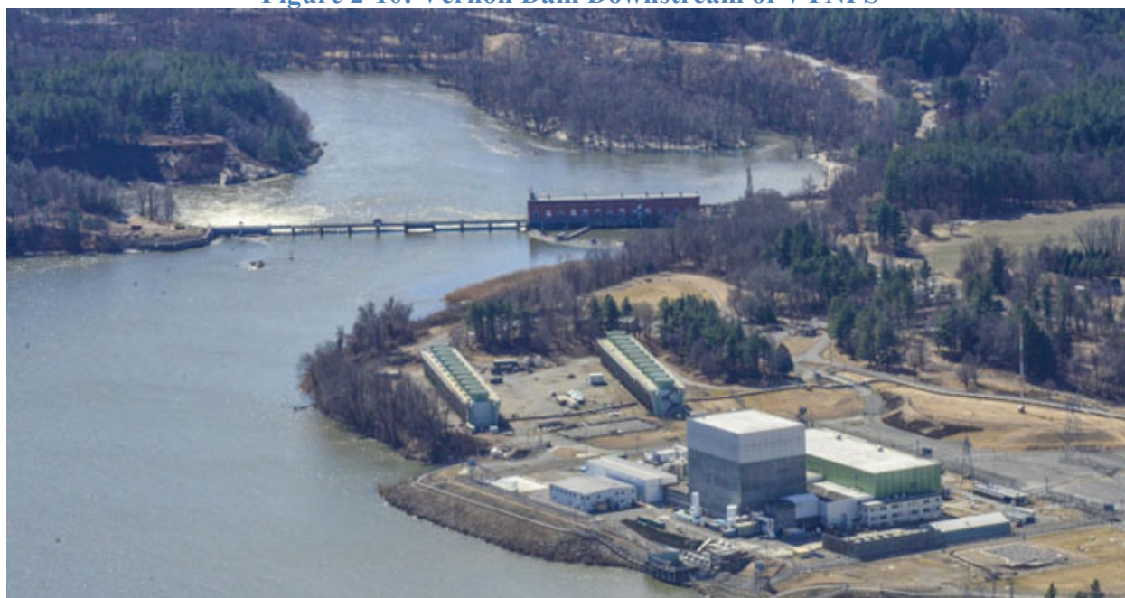
Figure 2-10: Vernon Dam Downstream of VYNPS
