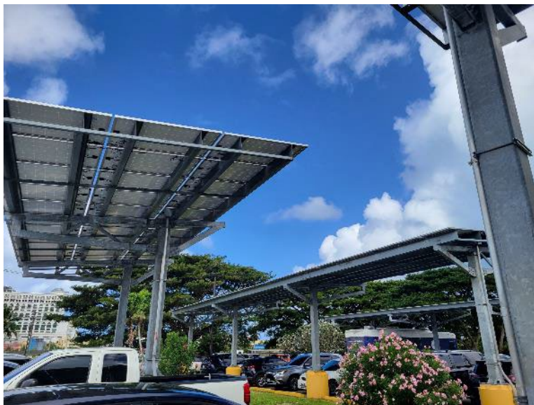
Figure 14. CHCC carport solar PV system.
