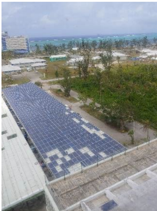
Figure 56. Damage from Typhoon Yutu to the solar PV system at the Marianas Business Plaza.
