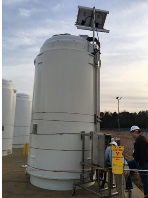
Figure 1. TN32B Cask in Storage (note: extra equipment is non-standard for data collection)
