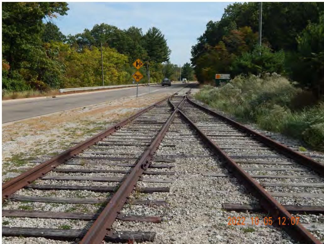
Figure 2-611. DC Cook Rail Spur Looking East
