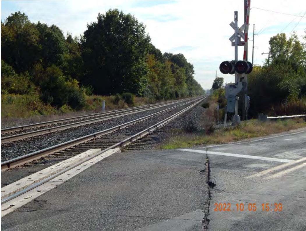
Figure 2-597. Aludyne Potential Transload Location Looking South
