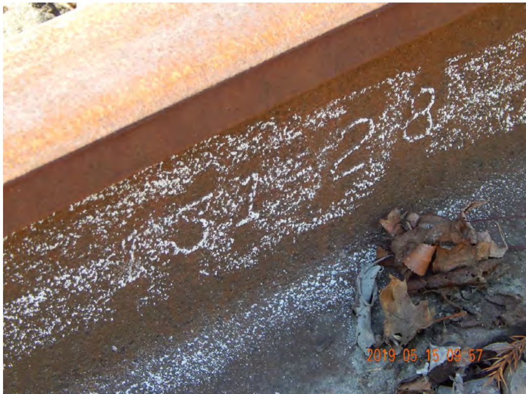
Figure 2-401. 131-lb. Rail at Morrisville Railyard (2019)
