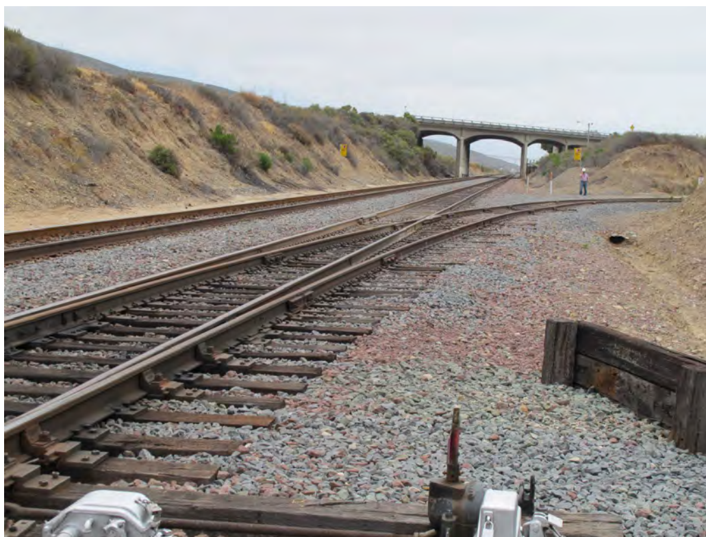
Figure 2-302. Mainline at San Onofre Site (Looking South) (2015)
