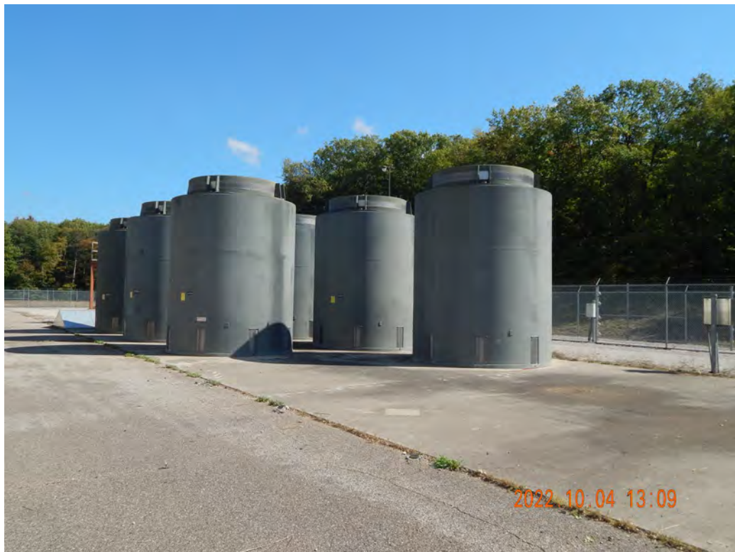
Figure 2-576. HI-STORM FW Dry Storage Systems at the East ISFSI at the Palisades Site
