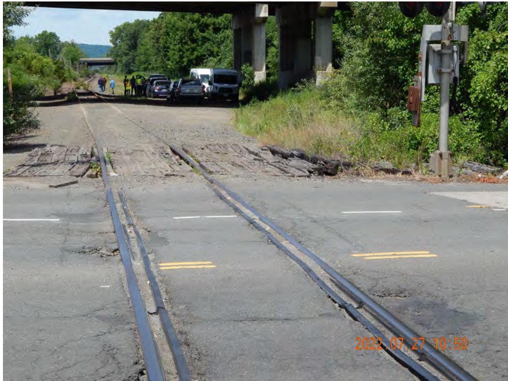
Figure 2-539. Segar Street Potential Transload Location Looking Northwest
