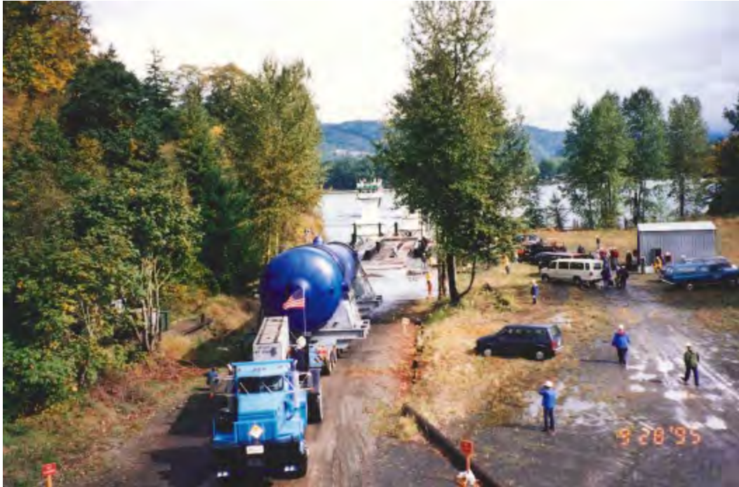
Figure 2-113. Trojan Steam Generator Being Loaded at Barge Slip (1995)
