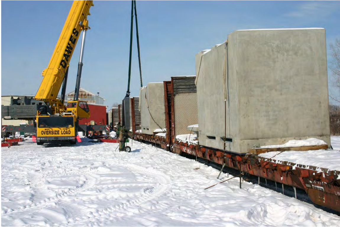
Figure 2-221. Horizontal Storage Module Transloading at Bellevue Location (2008)
