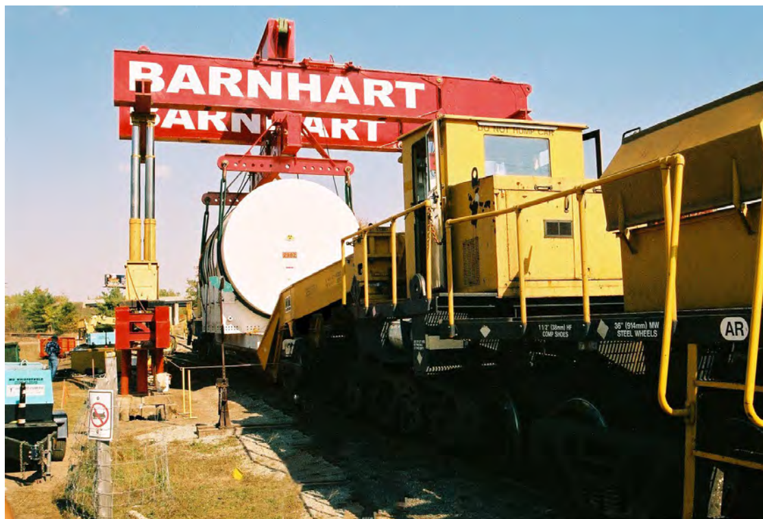
Figure 2-71. Transfer of Reactor Pressure Vessel onto ETMX1001 Railcar (2003)
