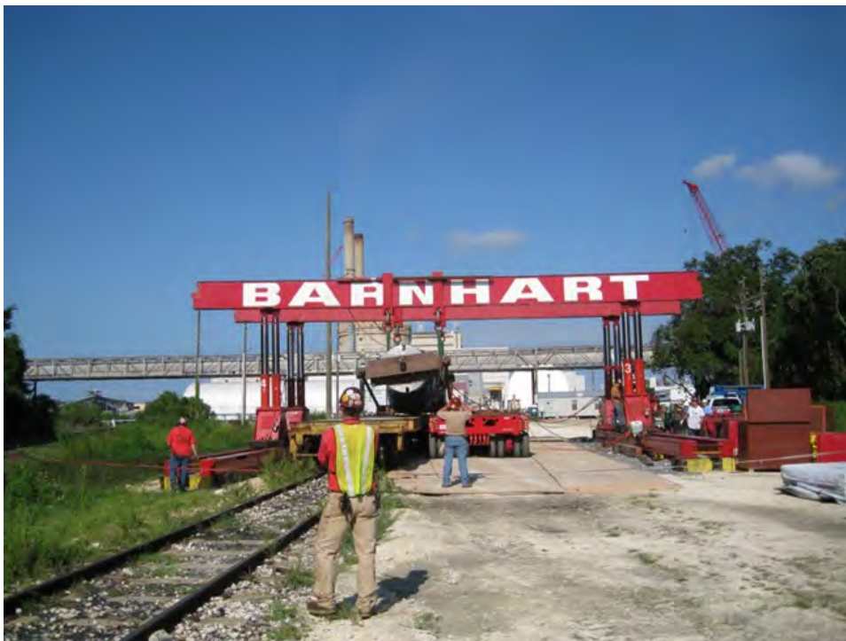
Figure 2-182. Generator Rotor Being Unloaded at the Crystal River Site (2009)
