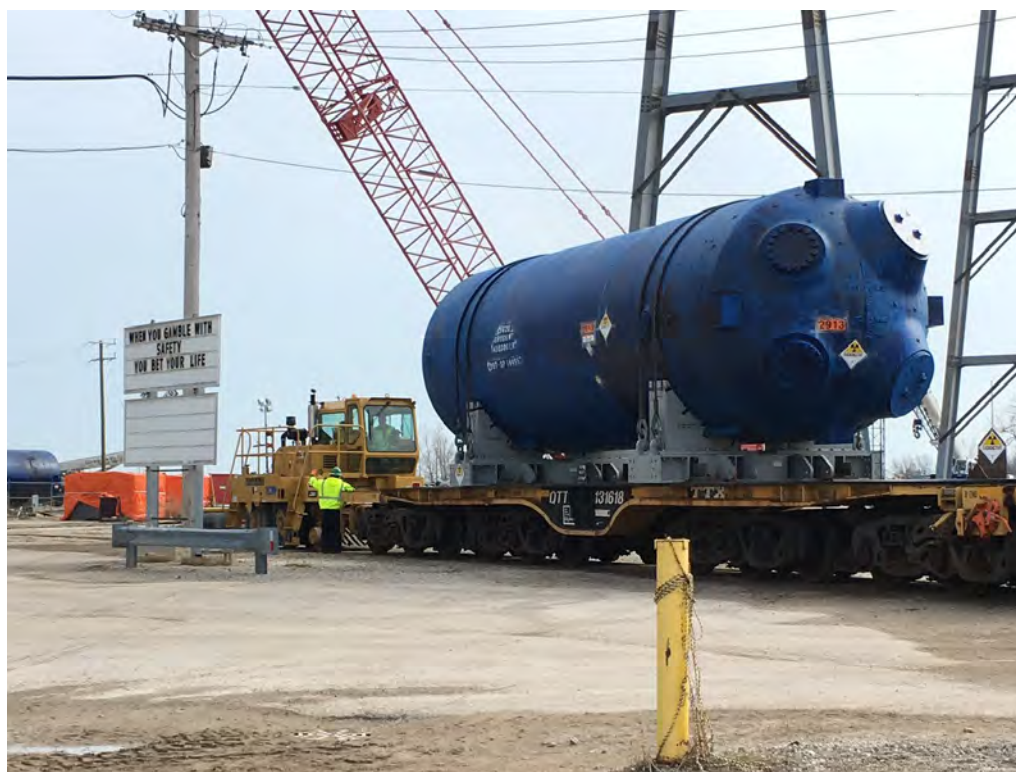
Figure 2-148. Steam Generator Being Prepared for Shipping (2016)
