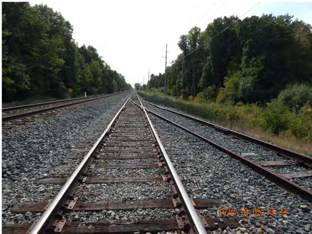
Figure 2-615. CSX Mainline at DC Cook Looking South
