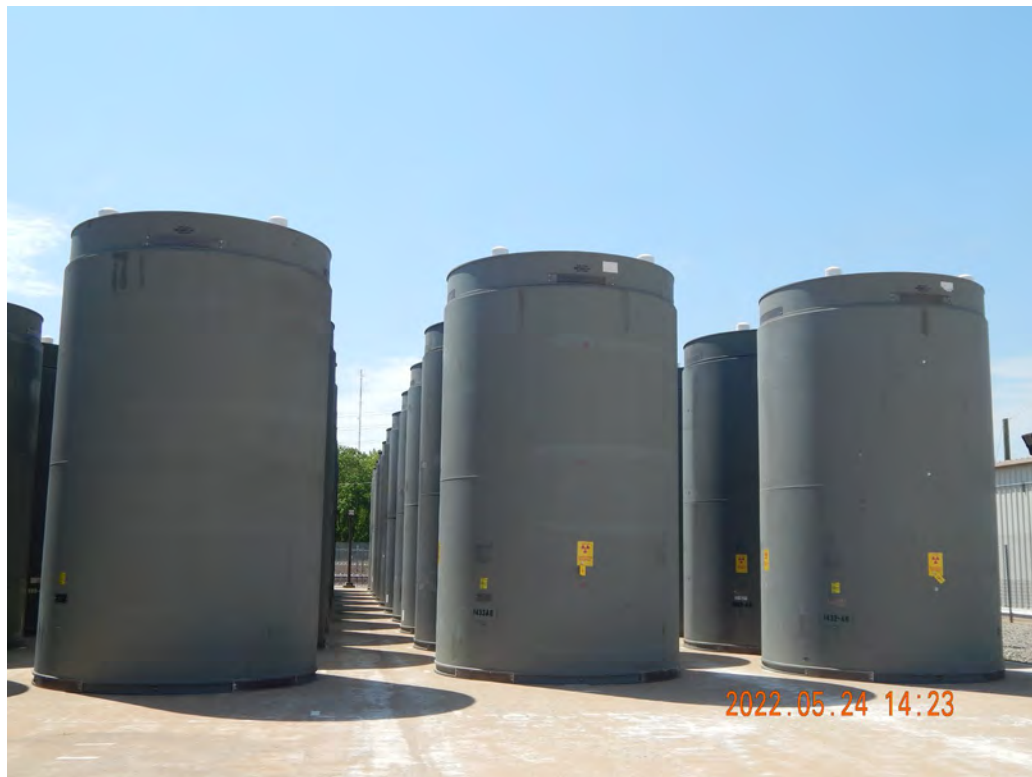
Figure 2-447. HI-STORM Dry Storage Systems at West ISFSI
