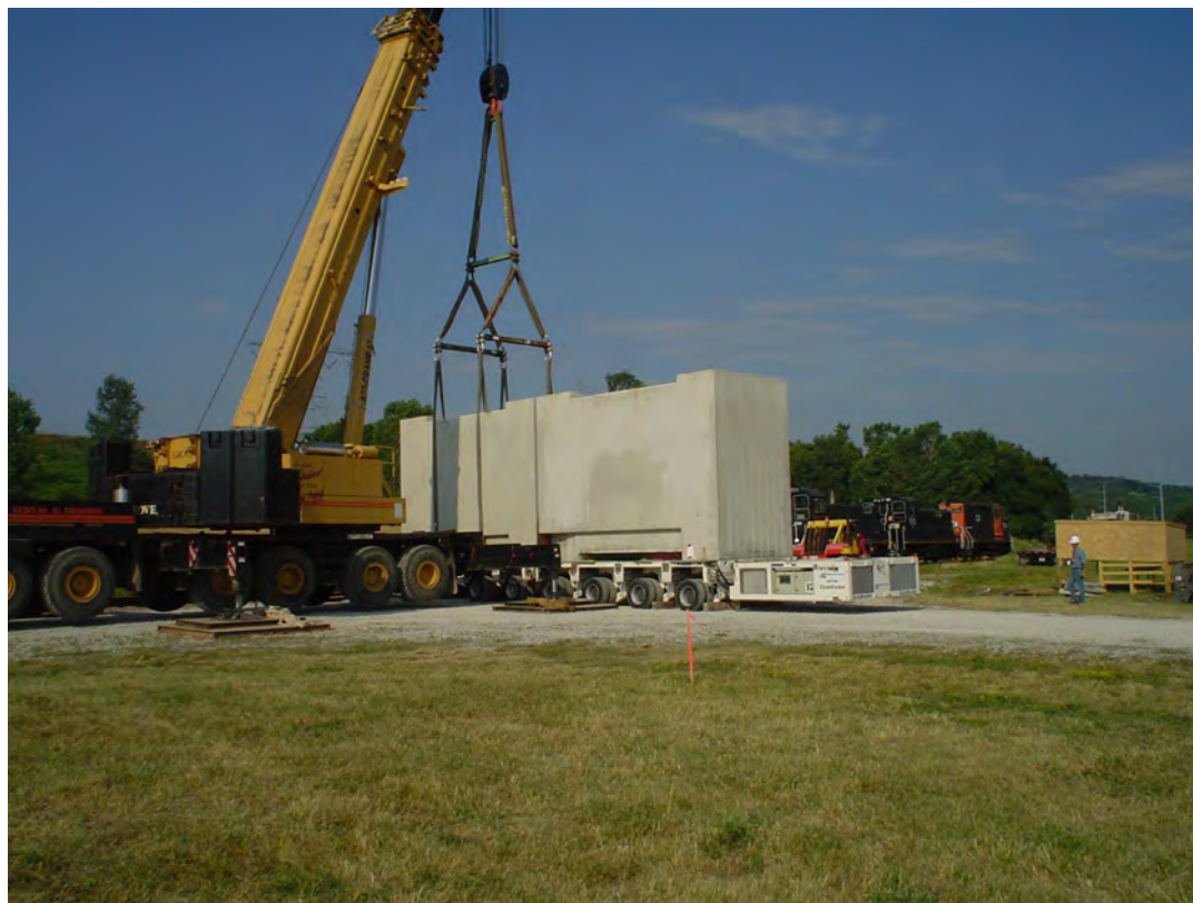
Figure 2-364. Horizontal Storage Module Being Transloaded from Railcar to Self-Propelled Modular Transporter
