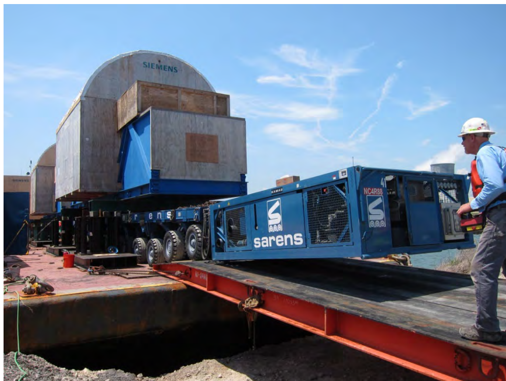
Figure 2-194. Turbine Components Being Unloaded Using Self-Propelled Modular Transporter (2012)
