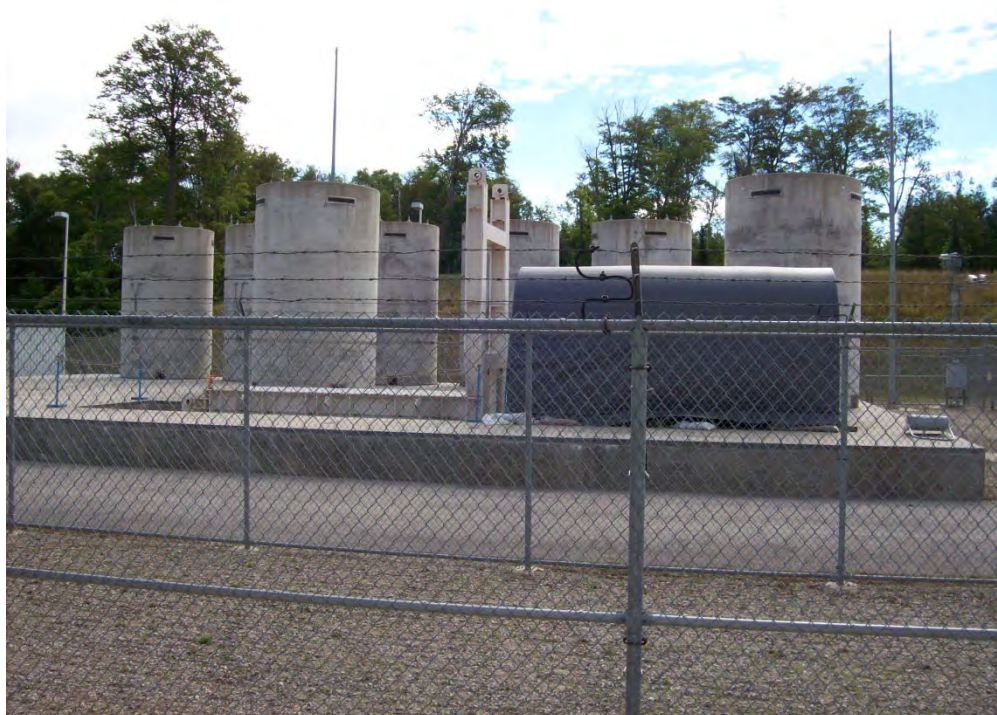
Figure 2-65. Transfer Cask and J-Skid at Big Rock Big Rock Point Independent Spent Fuel Storage Installation (2013)
