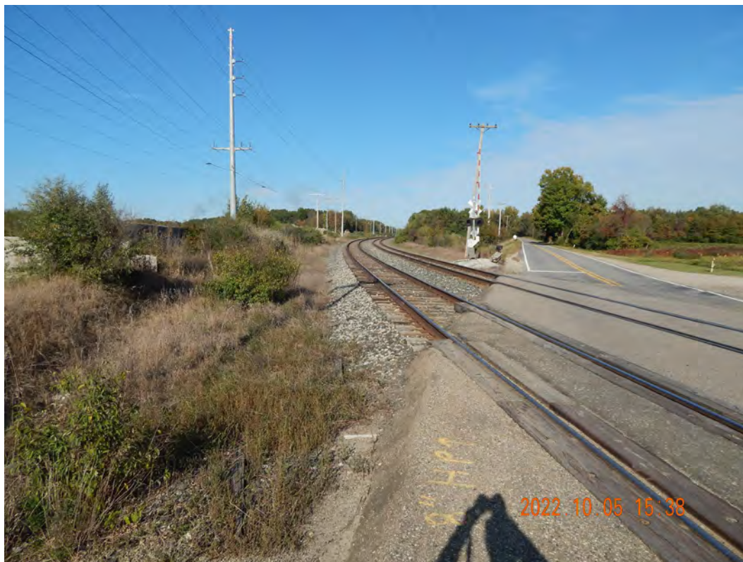
Figure 2-596. Quarry Potential Transload Location Looking North
