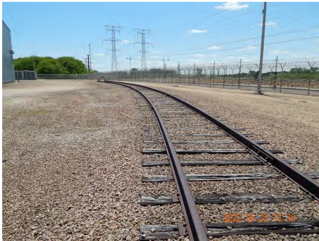
Figure 2-496. Western Rail Spur (Looking South)
