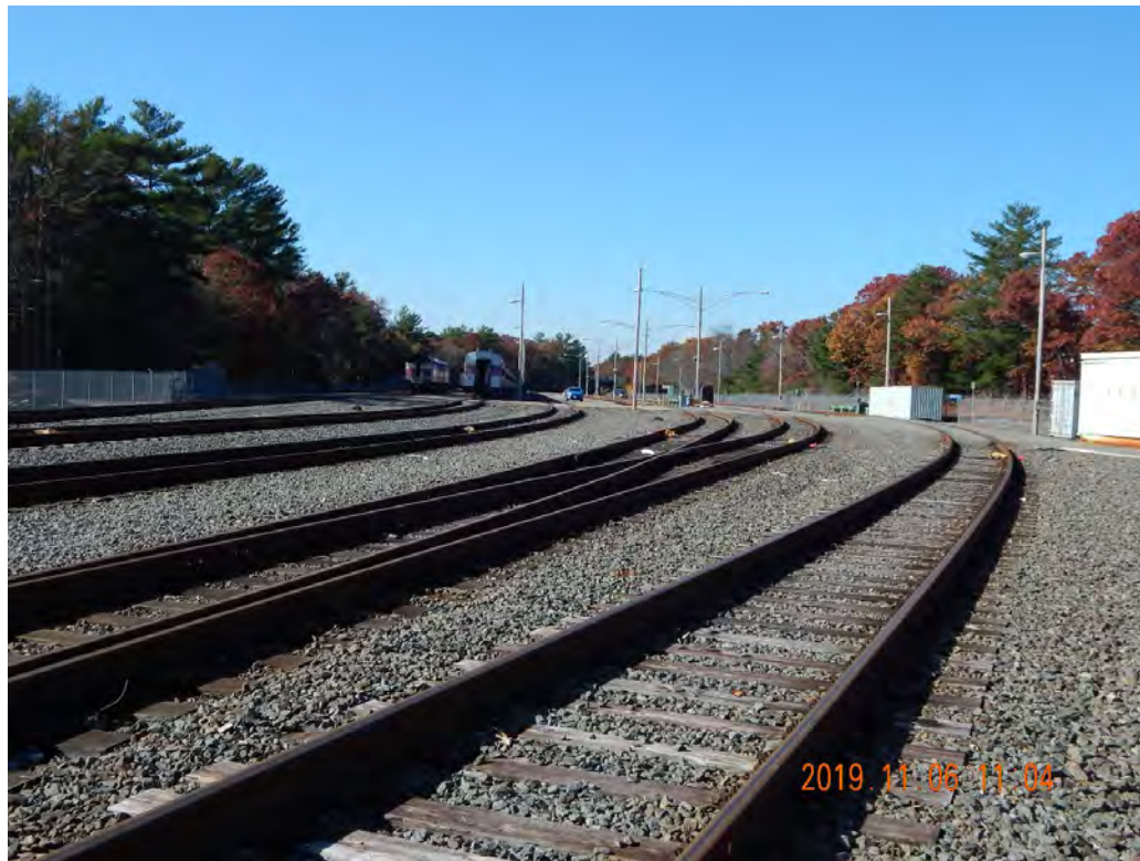
Figure 2-418. First Potential Rail Transload Location Looking West (2019)
