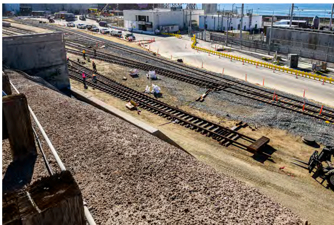
Figure 2-284. Expansion of On-site Rail Spur (Looking West) (2022)
