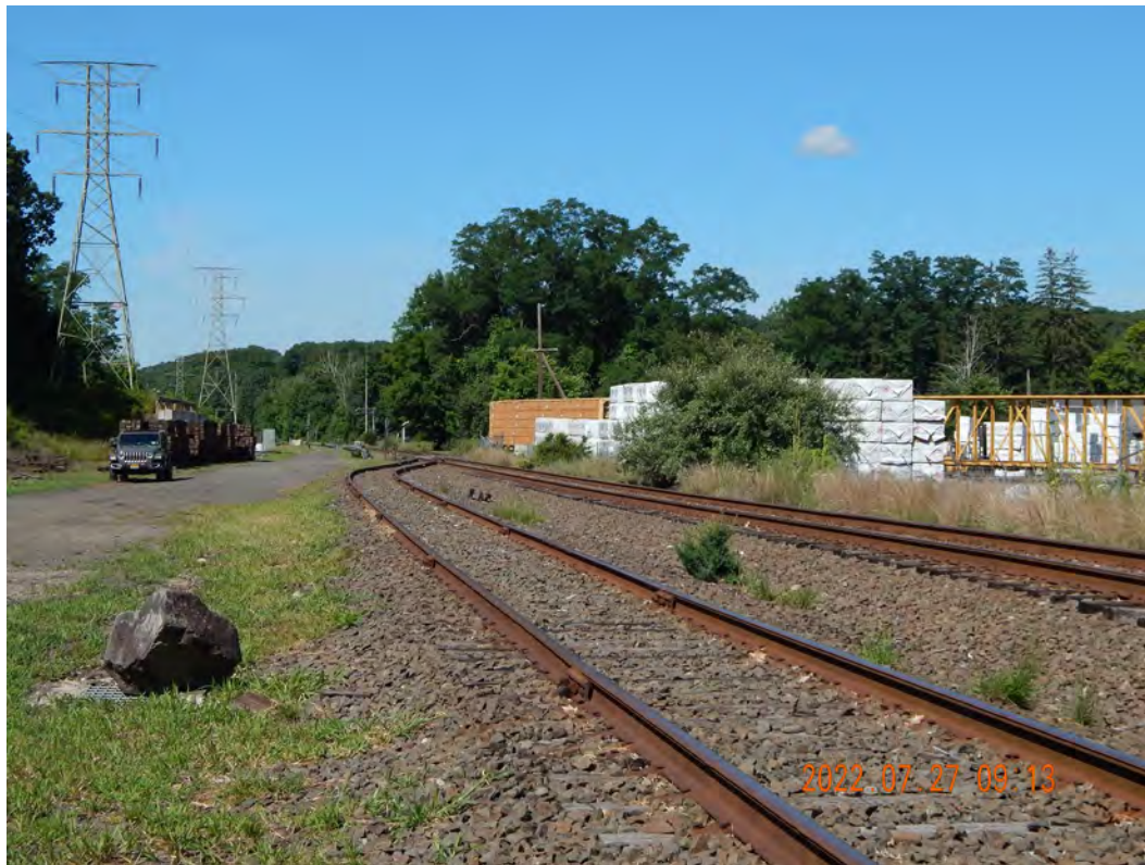
Figure 2-532. Hawleyville Road Potential Transload Location Looking Southwest
