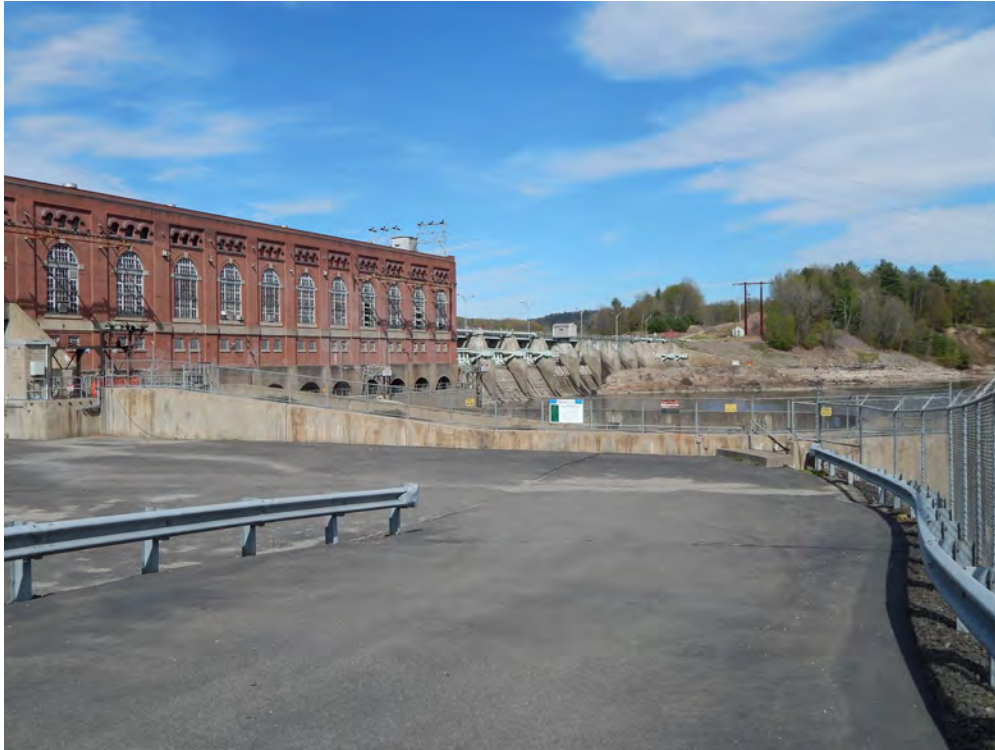
Figure 2-316. Vernon Dam and Hydroelectric Station (2016)
