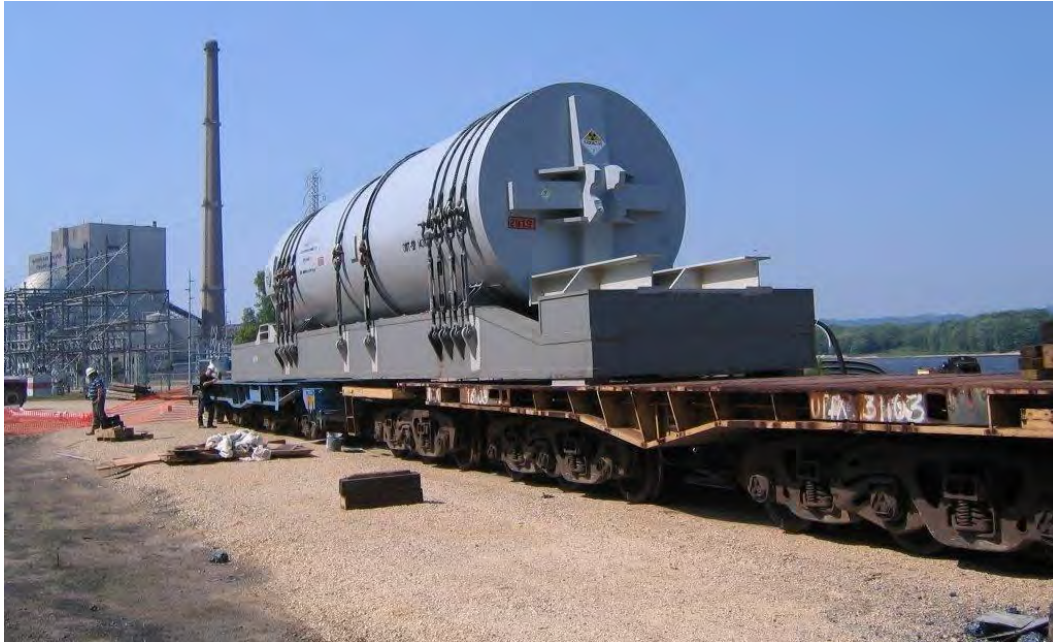
Figure 2-128. La Crosse Reactor Pressure Vessel on Rail Spur (2007)
