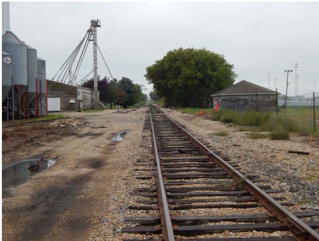
Figure 2-210. Potential Luxemburg Transload Location (Looking West) (2014)
