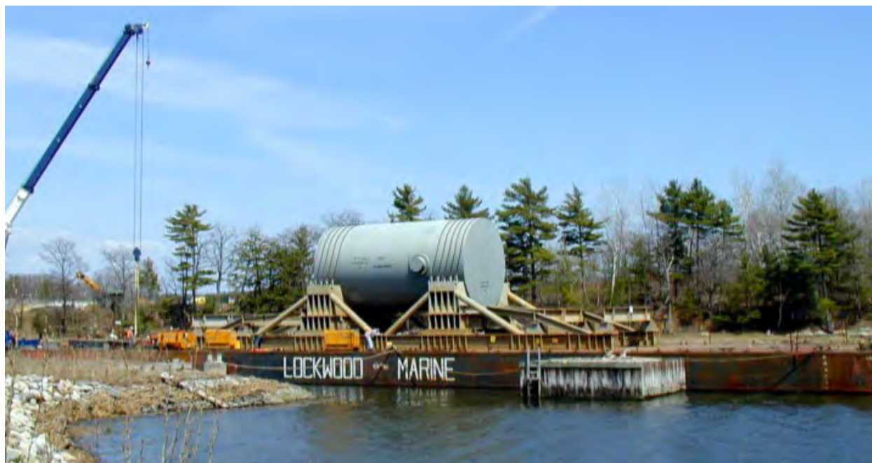
Figure 2-17. Maine Yankee Reactor Pressure Vessel Being Loaded onto Barge (2003)
