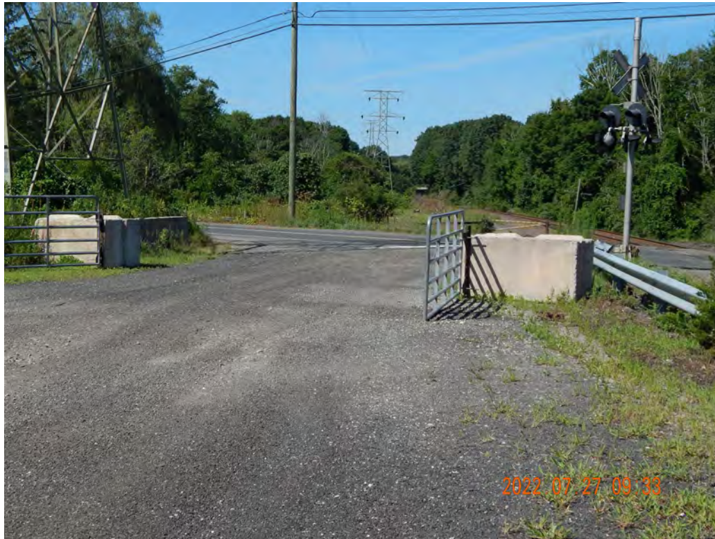
Figure 2-533. Hawleyville Road Entrance Looking Southwest
