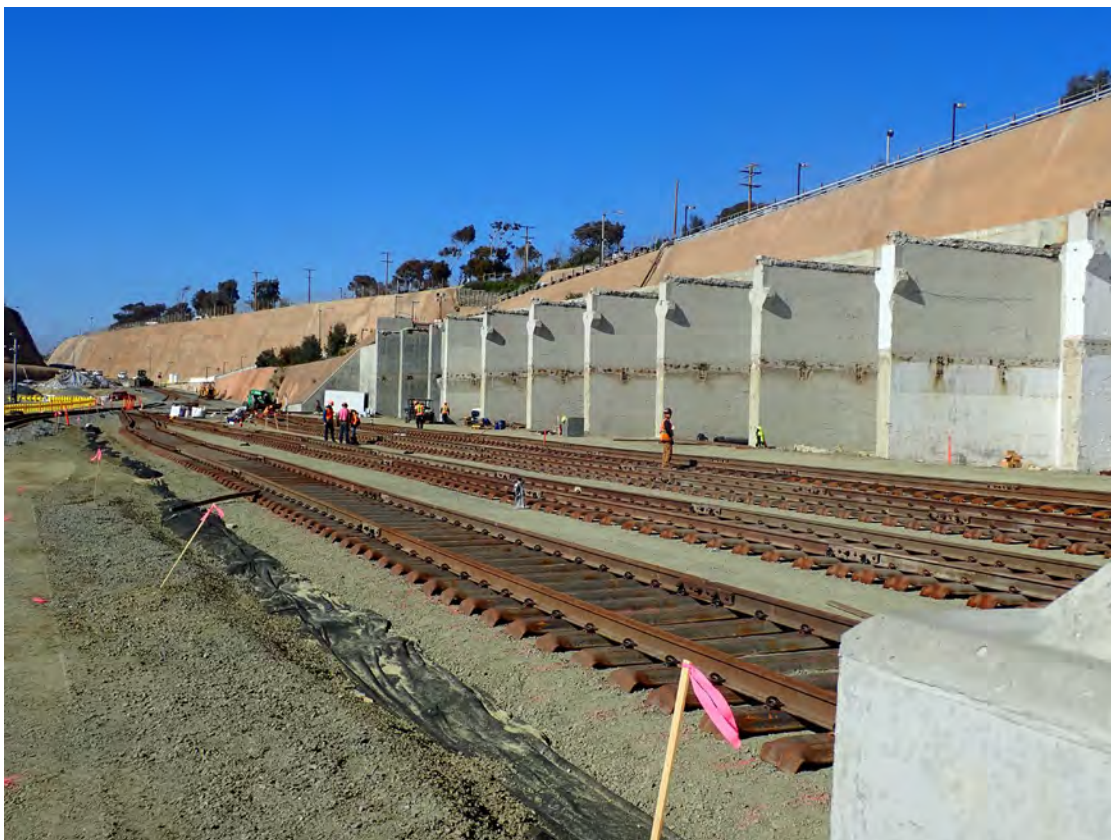
Figure 2-286. Expansion of On-site Rail Spur (Looking North) (2022)
