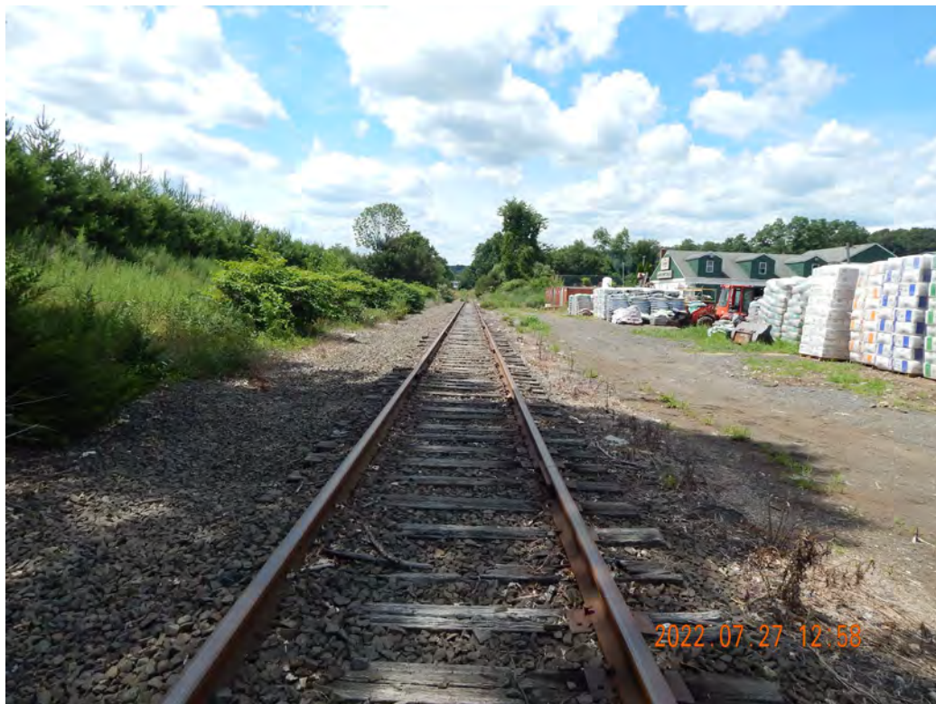
Figure 2-546. Agriventures Agway Potential Transload Location Looking Northwest
