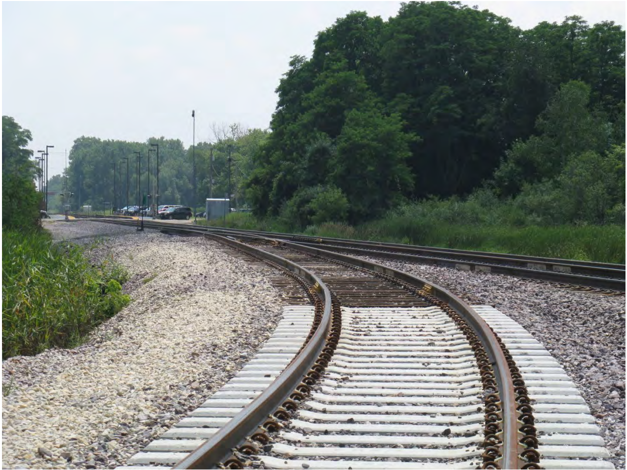
Figure 2-147. Junction of Zion On-site Rail Spur with Union Pacific Railroad Showing Concrete Rail Ties (2013)
