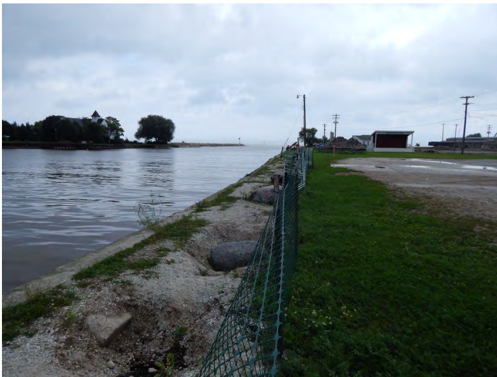
Figure 2-249. Potential Kewaunee Barge Transload Location Water Front (2014)
