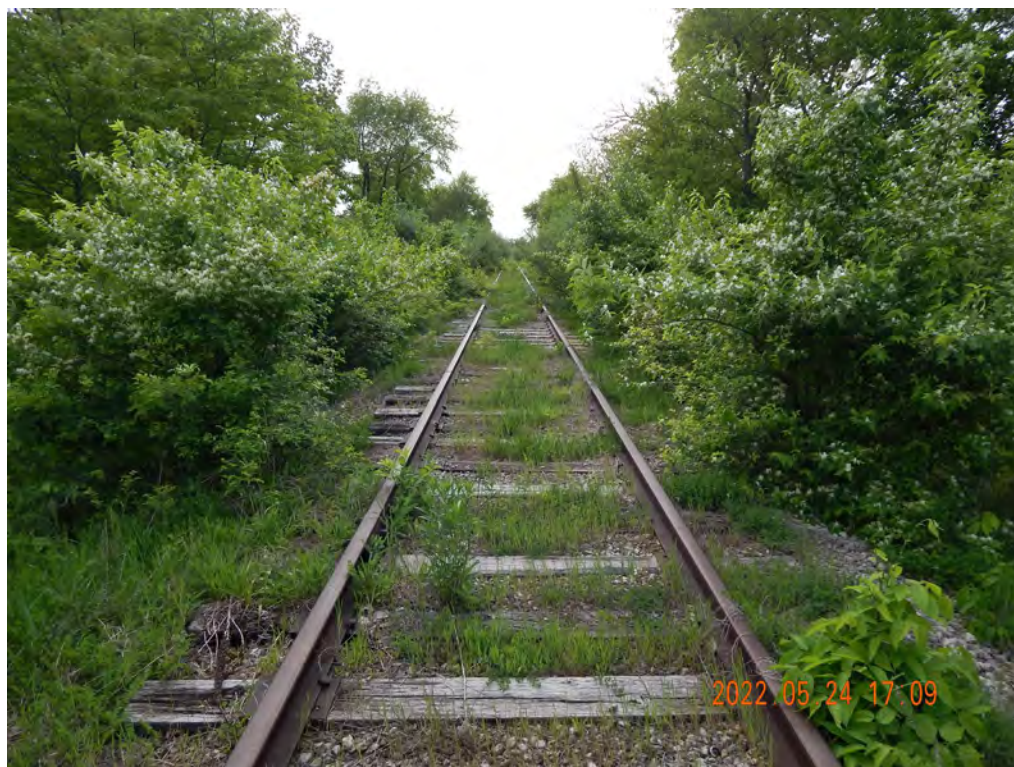
Figure 2-454. Rail Spur at Lock Road Looking West
