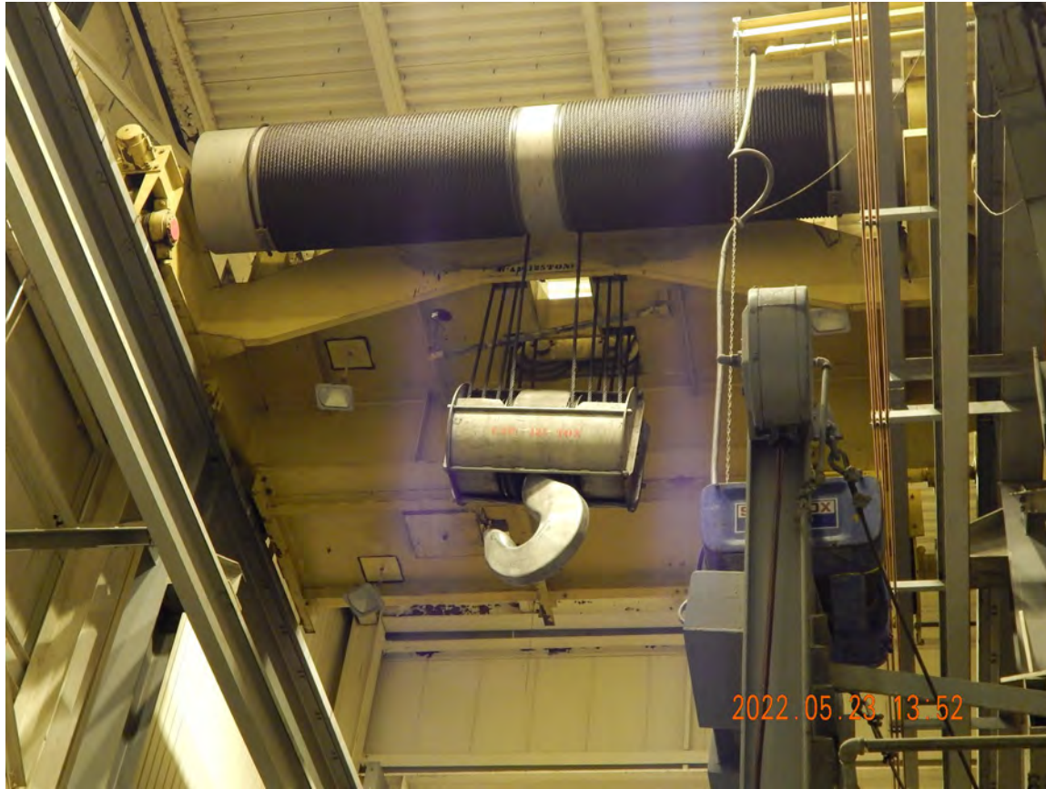
Figure 2-484. 125-Ton Crane at the Morris Site
