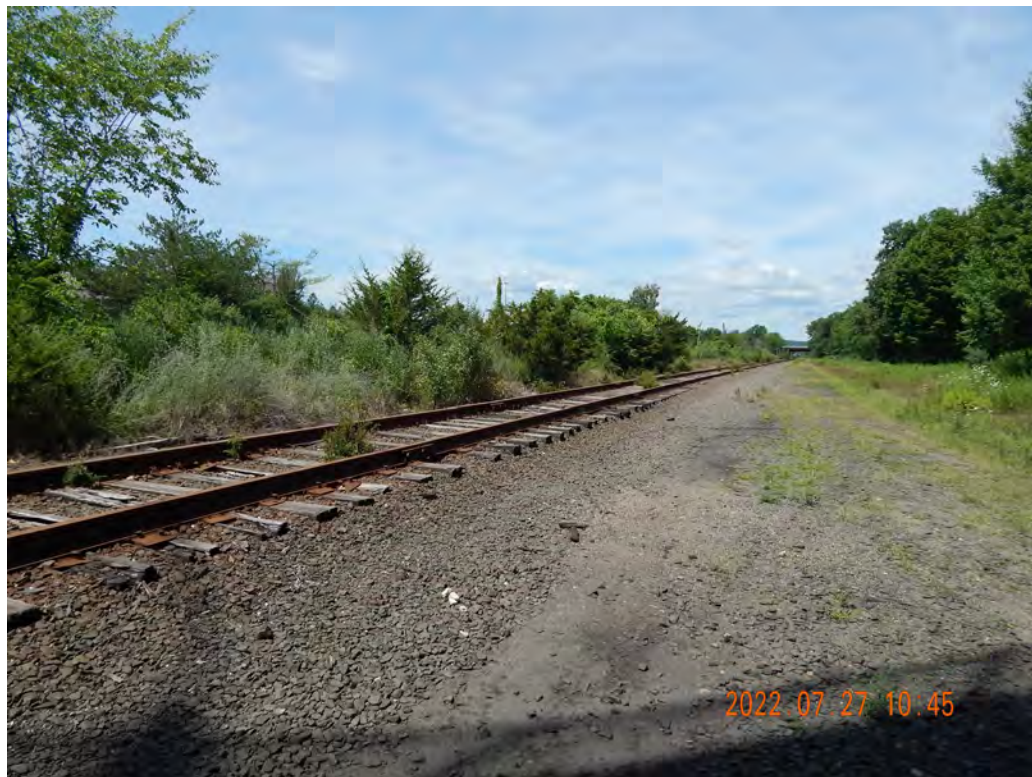
Figure 2-542. Segar Street Potential Transload Location Looking Northwest
