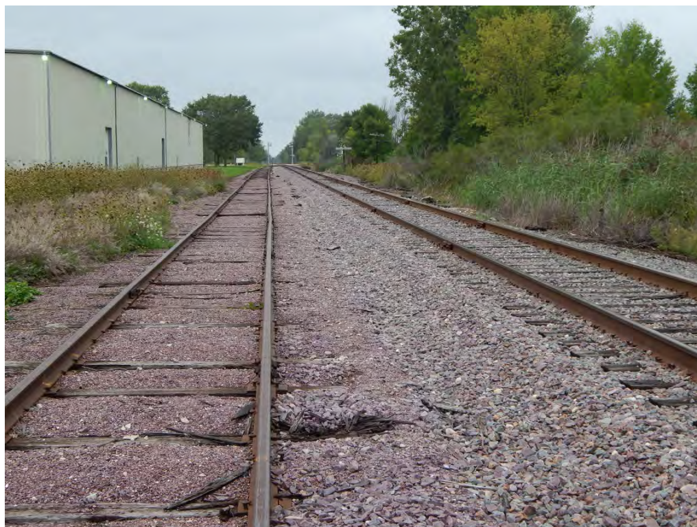
Figure 2-217. Potential Bellevue Transload Location (Looking North) (2014)
