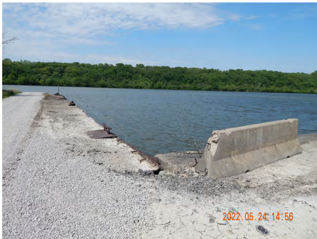
Figure 2-471. Dresden Barge Area Looking North
