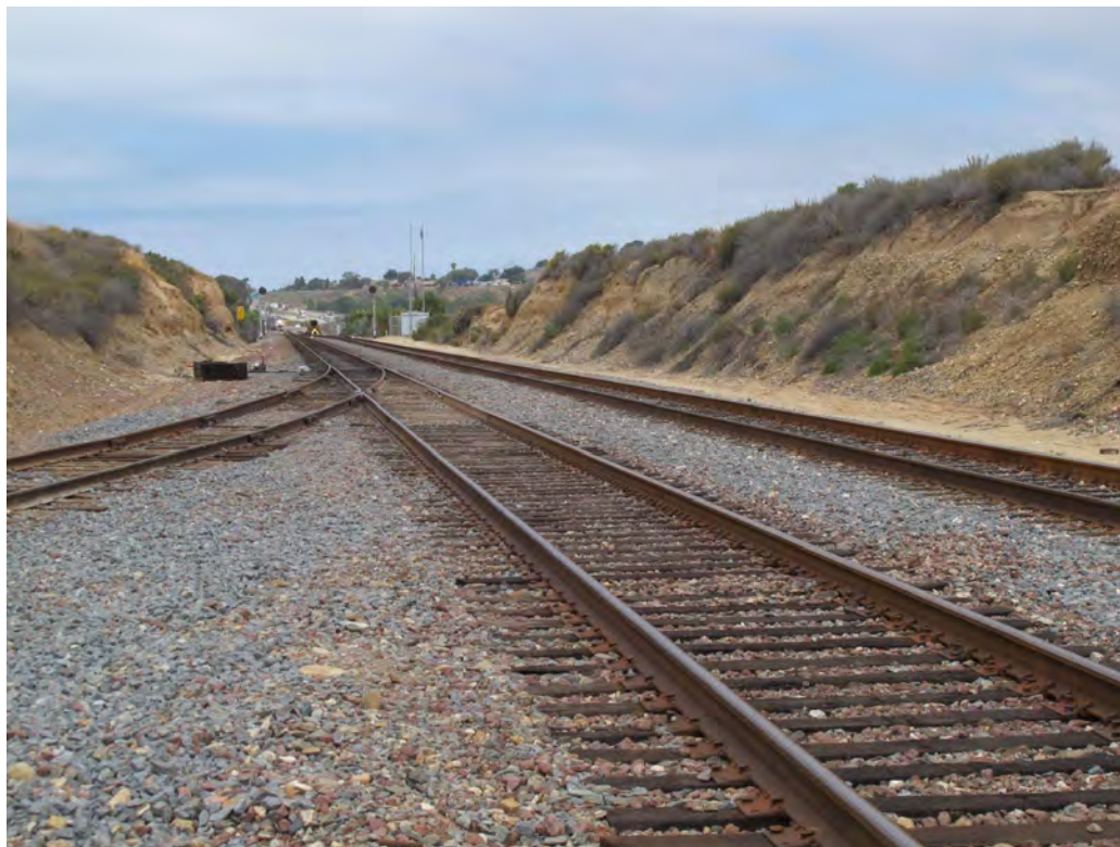
Figure 2-301. Mainline at San Onofre Site (Looking North) (2015)
