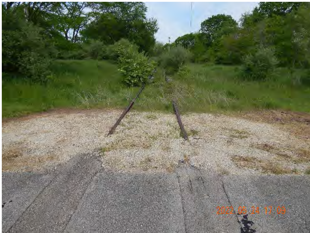
Figure 2-453. Rail Spur at Lock Road Looking East
