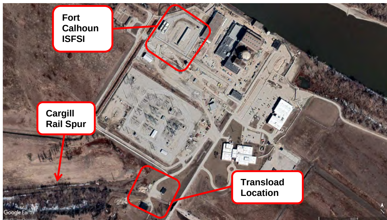
Figure 2-363. Aerial View of Transload Location (Google 2022)
