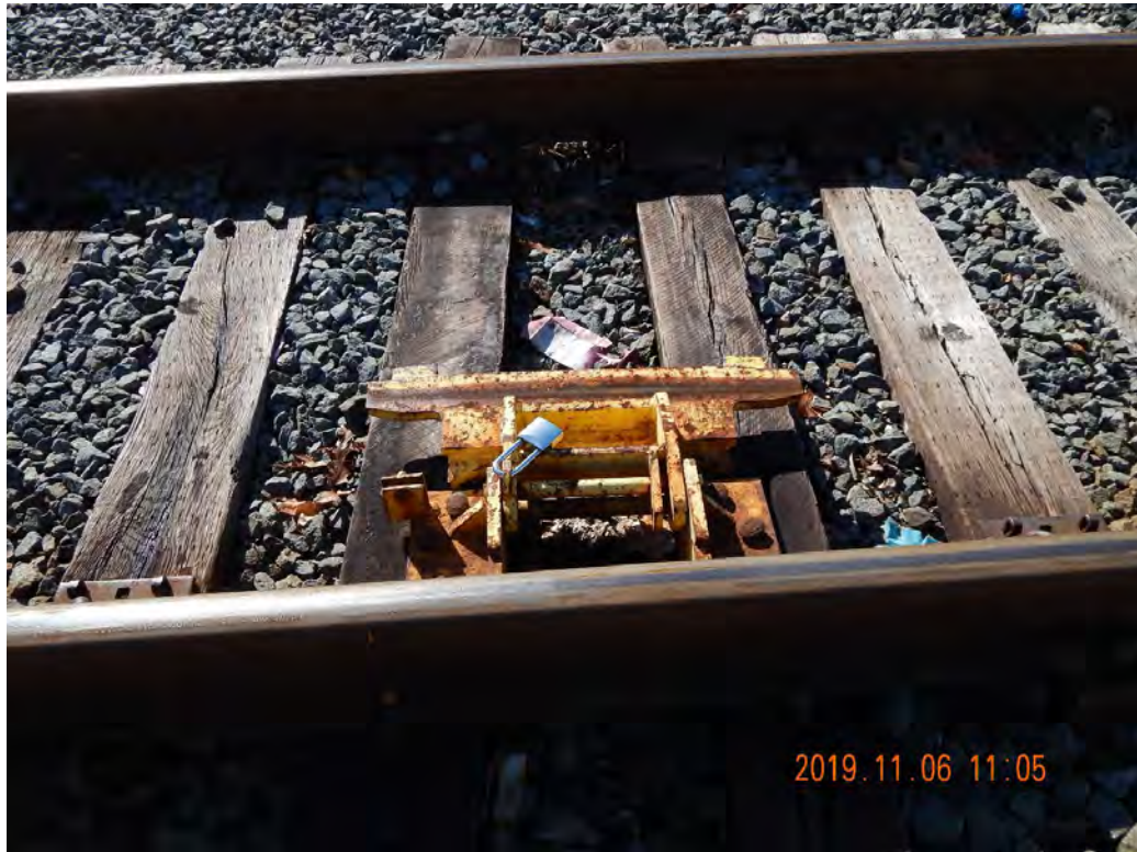
Figure 2-419. Derailer at First Potential Rail Transload Location (2019)
