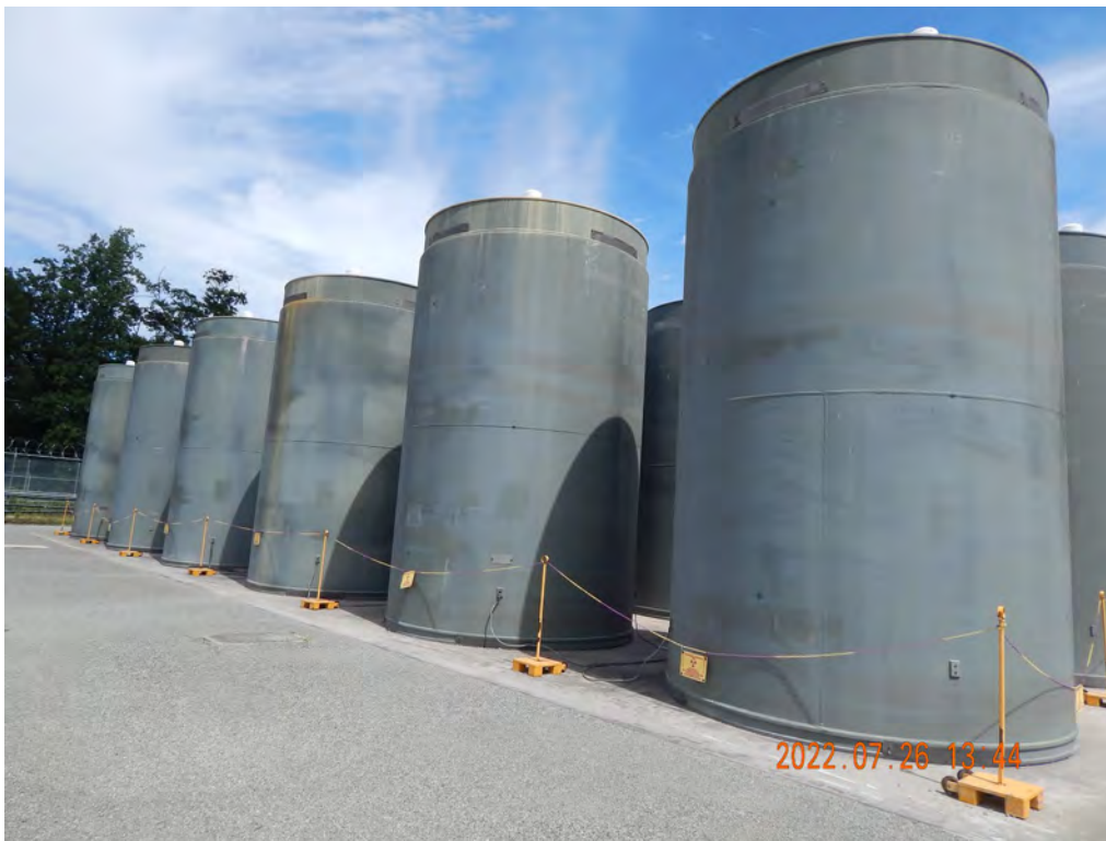
Figure 2-512. HI-STORM FW Dry Storage Systems at the Indian Point ISFSI (Looking North)
