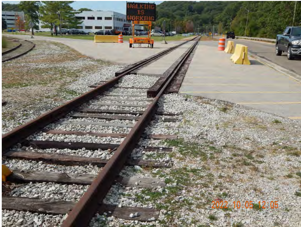
Figure 2-610. DC Cook Rail Spur Looking West
