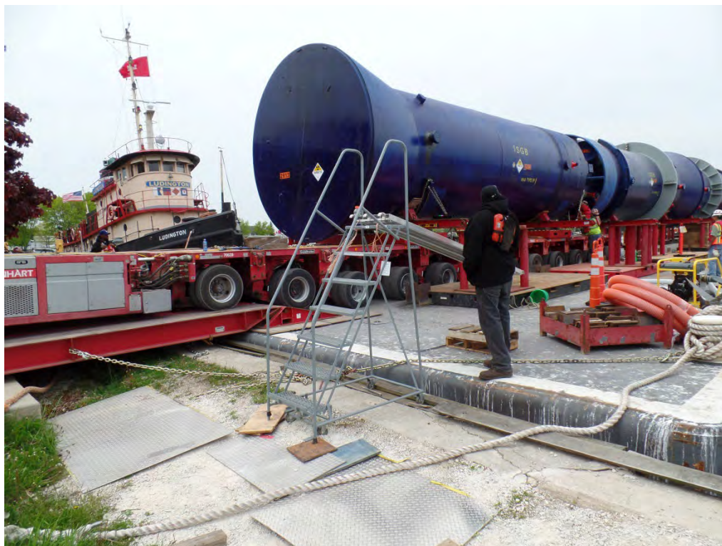
Figure 2-255. Fourth Steam Generator Moving onto Barge (2014)
