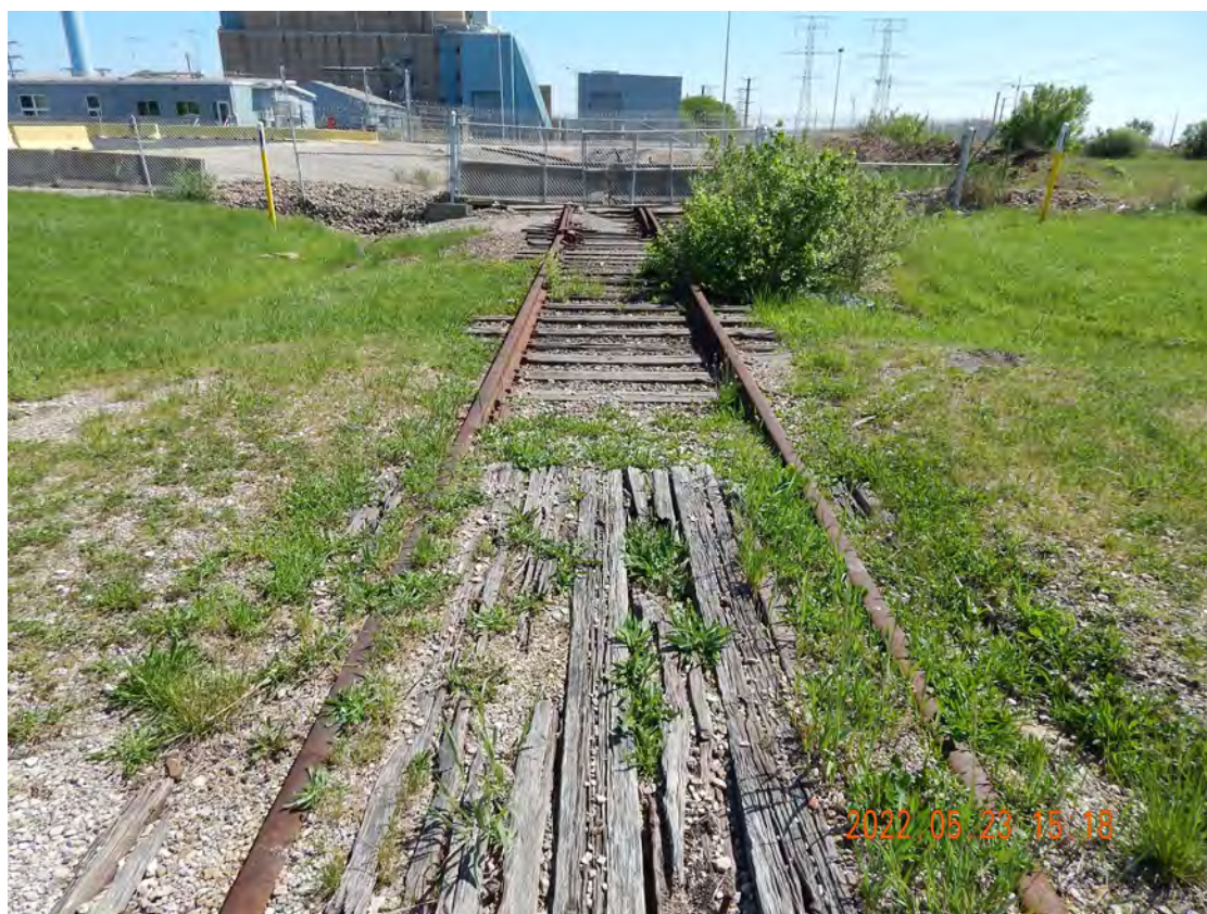
Figure 2-500. Morris Rail Spur Approaching the Morris Site
