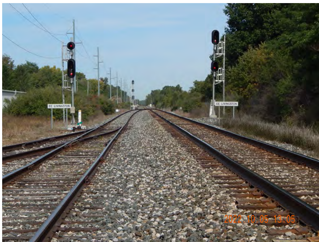
Figure 2-616. CSX Mainline at DC Cook Looking North
