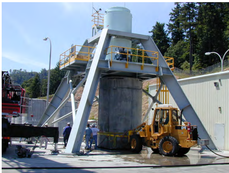
Figure 2-105. Trojan Transfer Station with Transfer Cask and TranStor Vertical Concrete Storage Overpack
