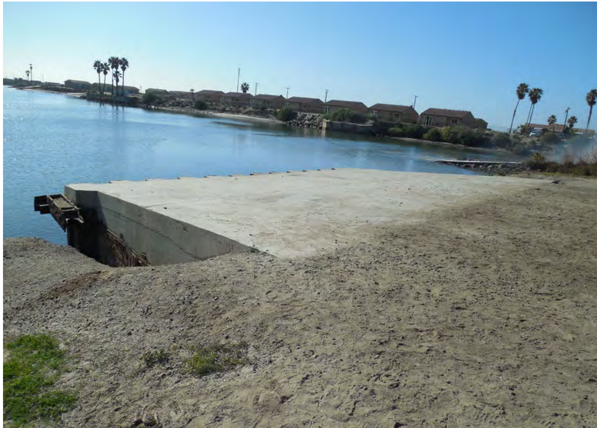
Figure 2-311. Del Mar Boat Basin Bulkhead (2016)
