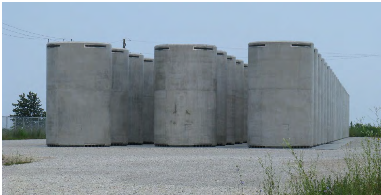
Figure 2-139. Vertical Concrete Storage Casks Staged at Zion (2013)
