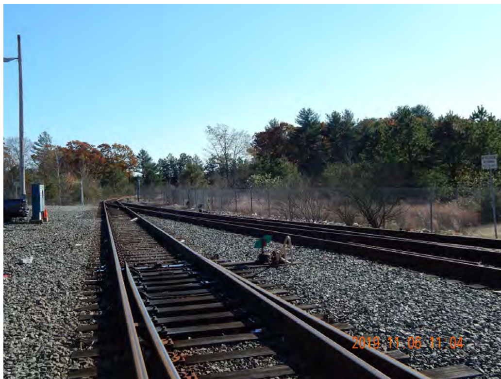
Figure 2-417. First Potential Rail Transload Location Looking East (2019)
