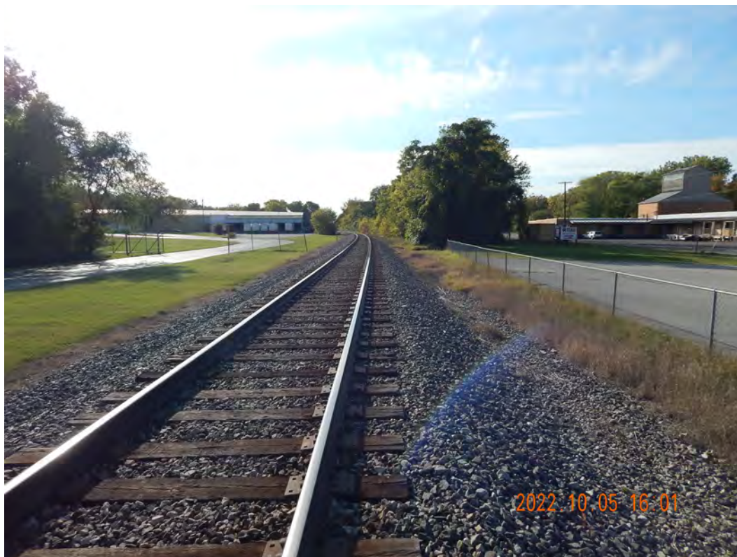
Figure 2-605. Menasha Packaging Potential Transload Location Looking West
