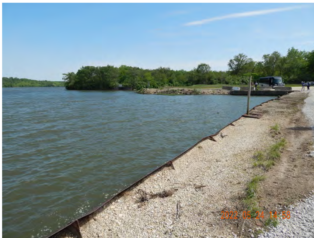
Figure 2-472. Dresden Barge Area Looking South
