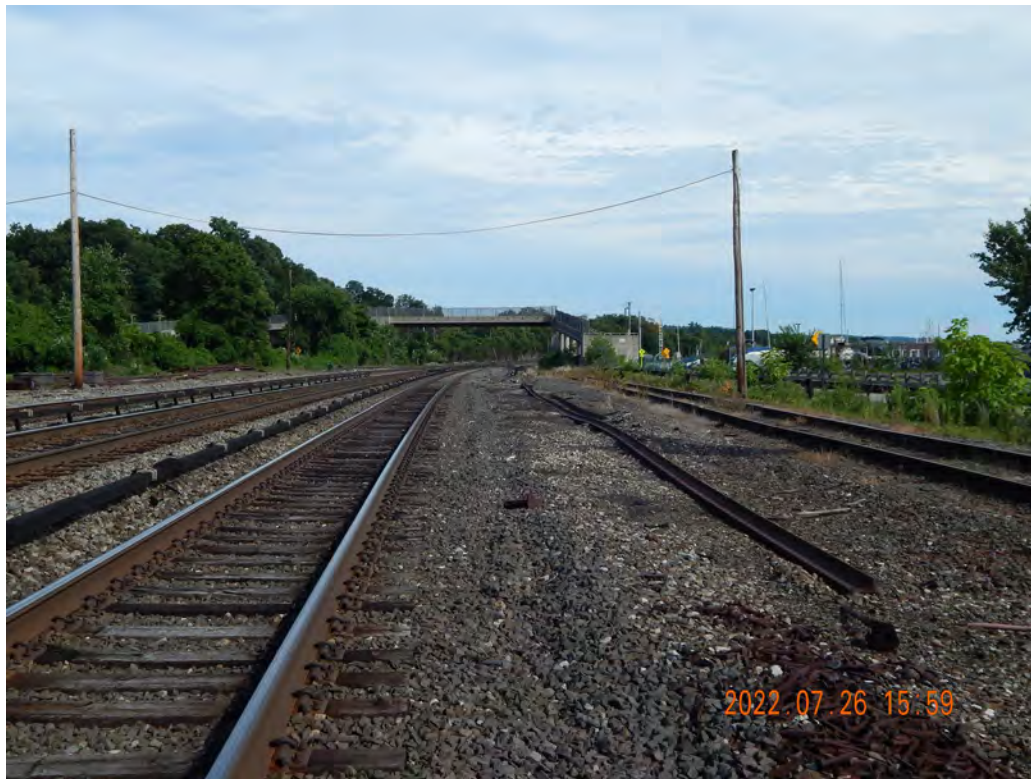
Figure 2-557. Croton Railyard Potential Transload Location Looking Southeast
