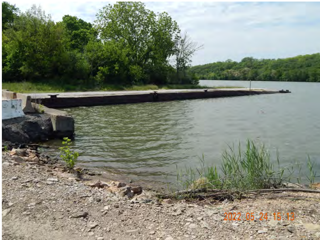
Figure 2-473. Dresden Barge Area Looking Northwest
