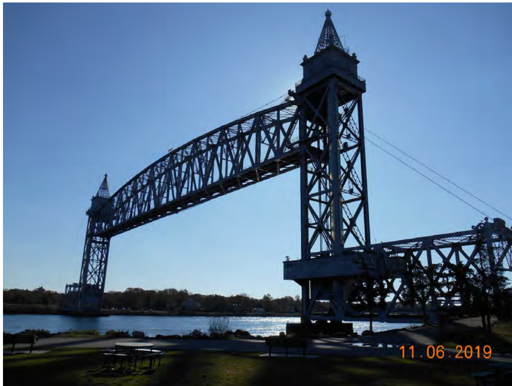
Figure 2-438. Cape Cod Canal Railroad Bridge (2019)
