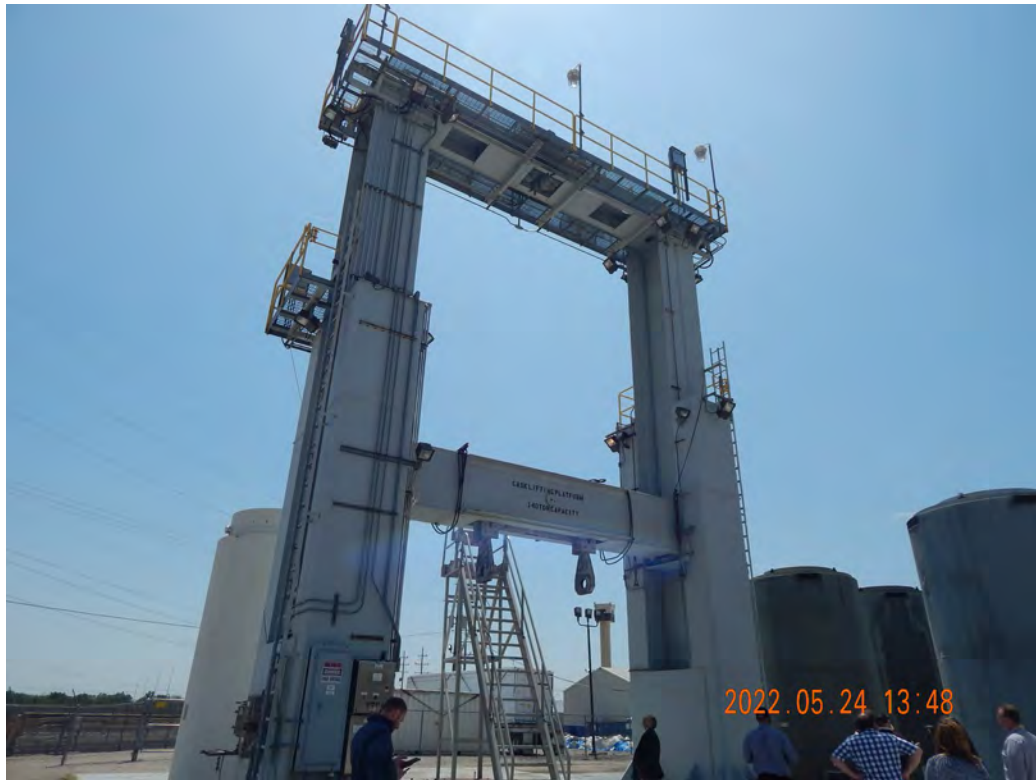
Figure 2-448. Cask Lifting Platform at Dresden Site
