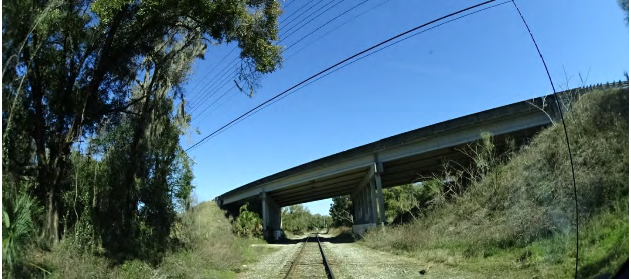
Figure 2-171. Highway Bridge over Florida Northern Railroad (2015)
