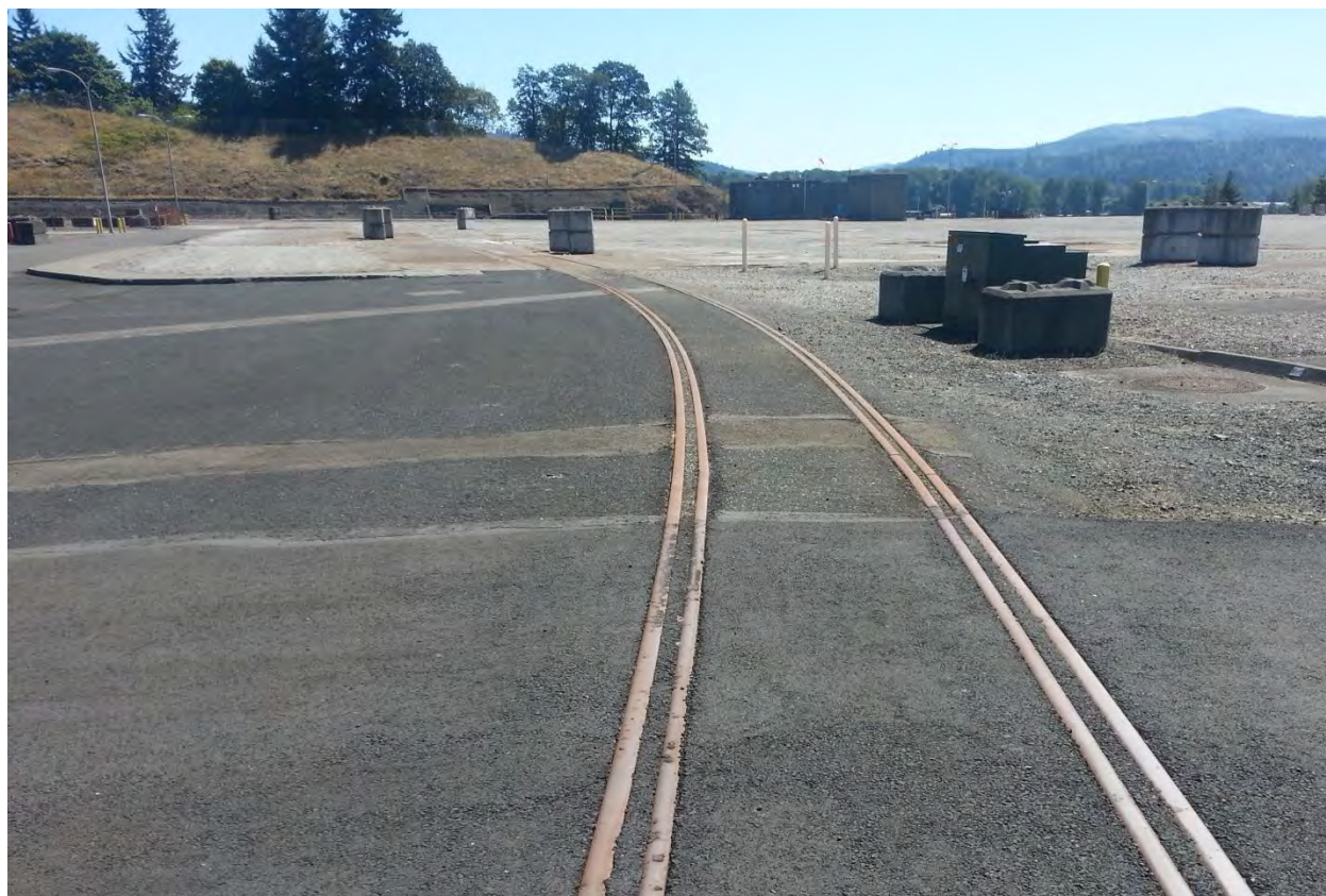
Figure 2-110. Remnants of On-site Rail Spur at Trojan (2013)
