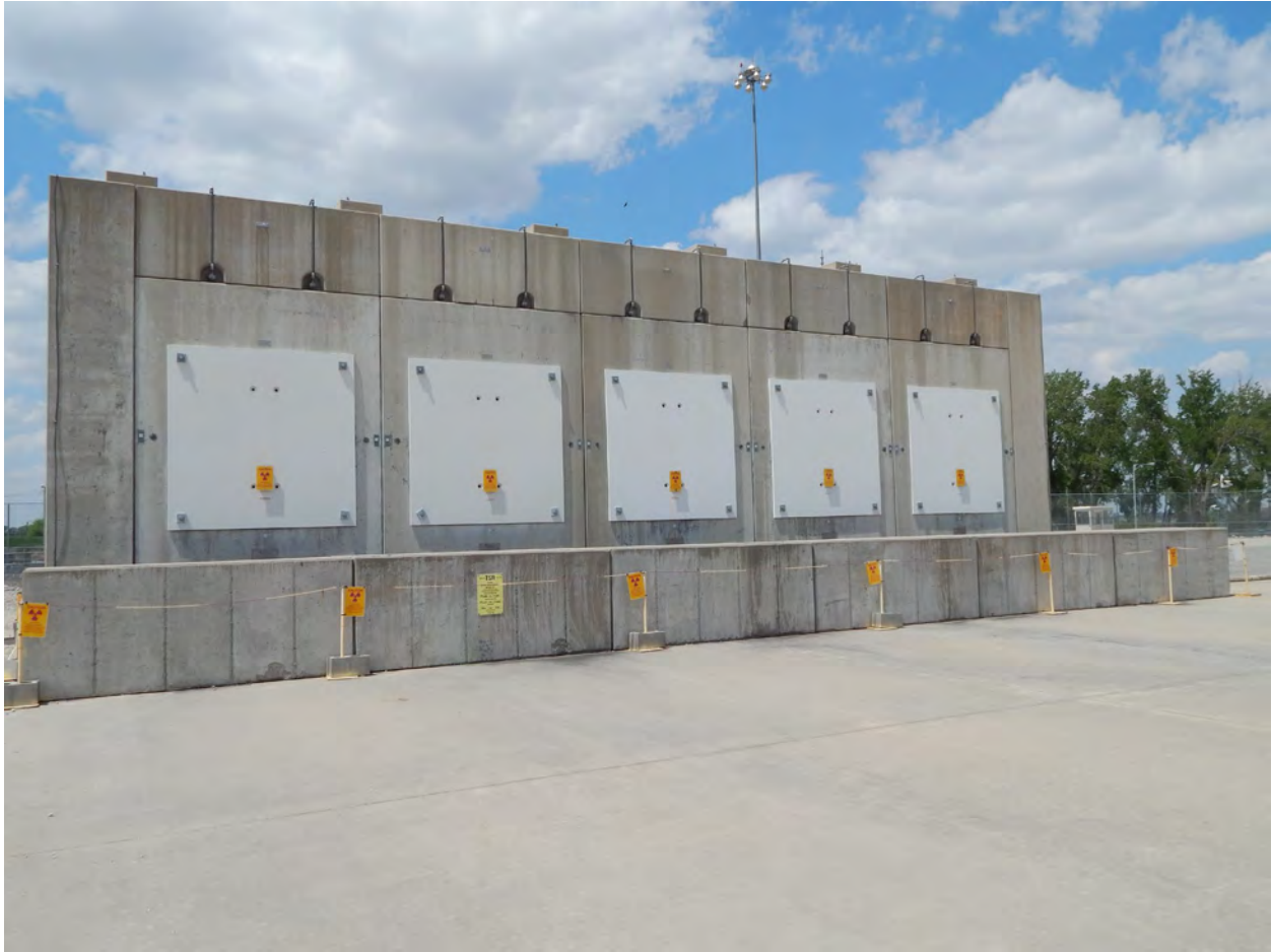
Figure 2-345. Fort Calhoun Independent Spent Fuel Storage Installation (2017)
