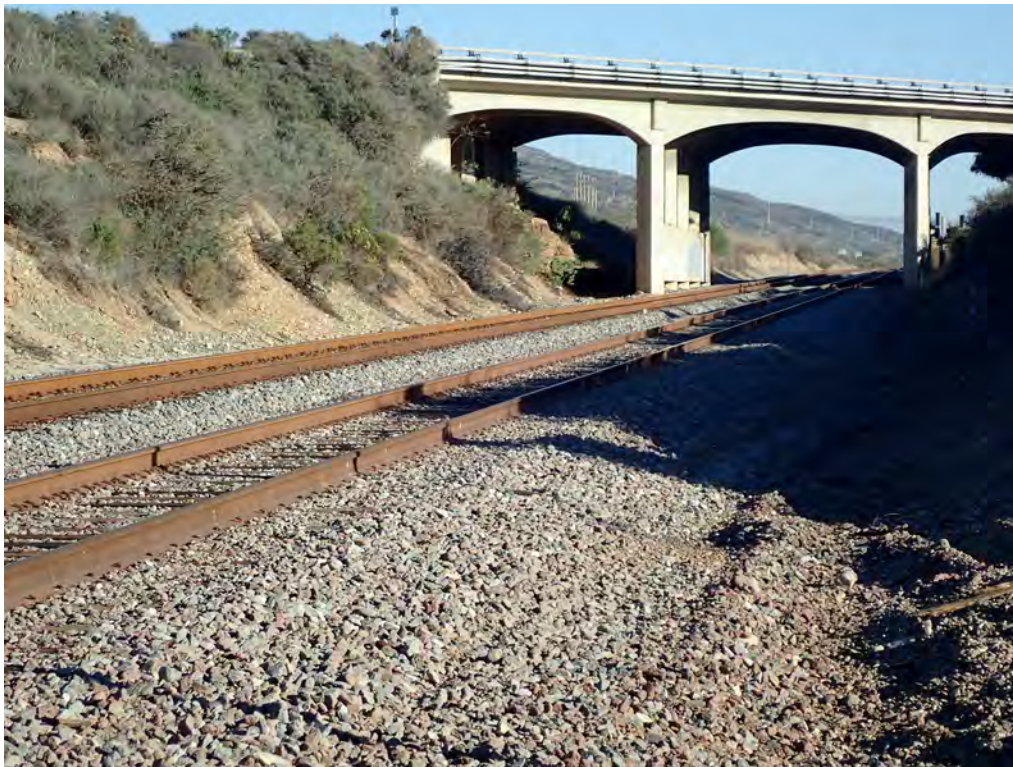
Figure 2-294. BNSF Mainline Looking South (2022)
