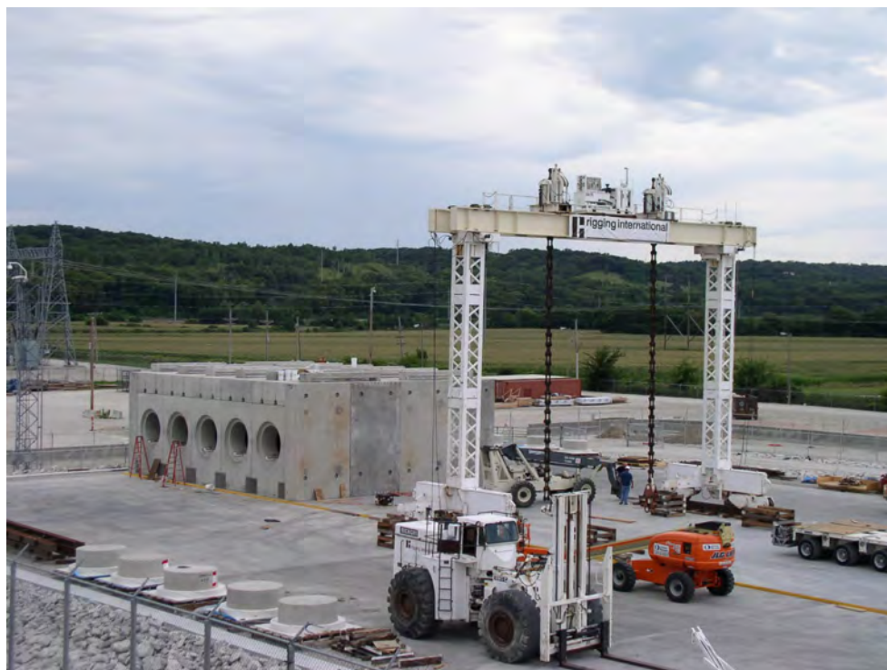
Figure 2-366. Installation of Horizontal Storage Modules at Independent Spent Fuel Storage Installation
