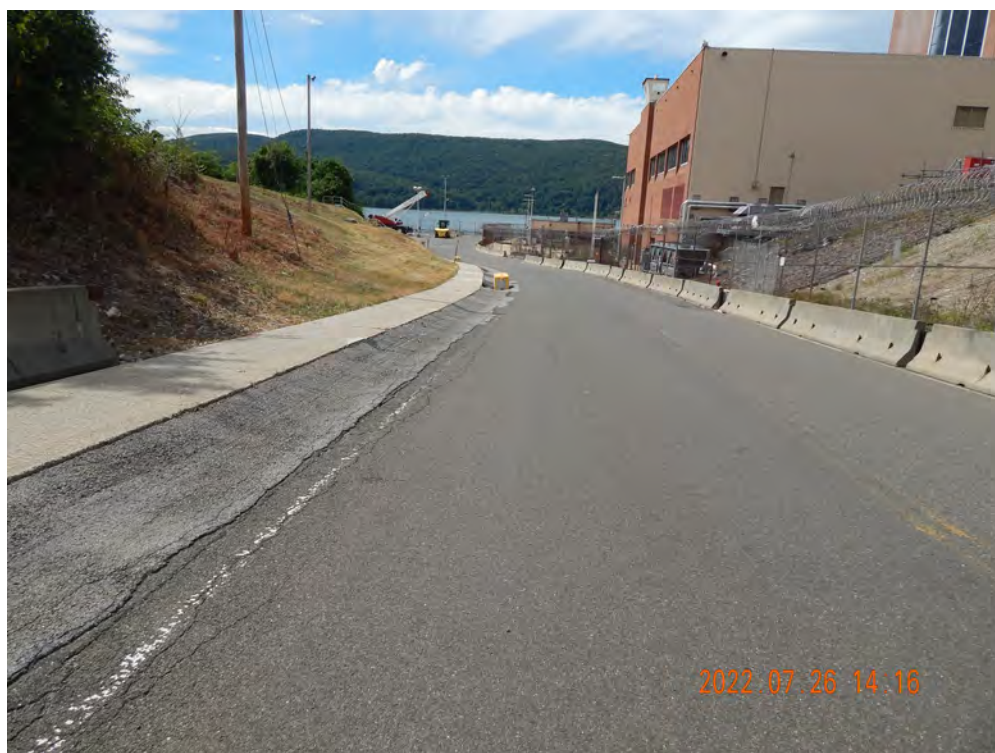
Figure 2-523. Indian Point Barge Area Access Road
