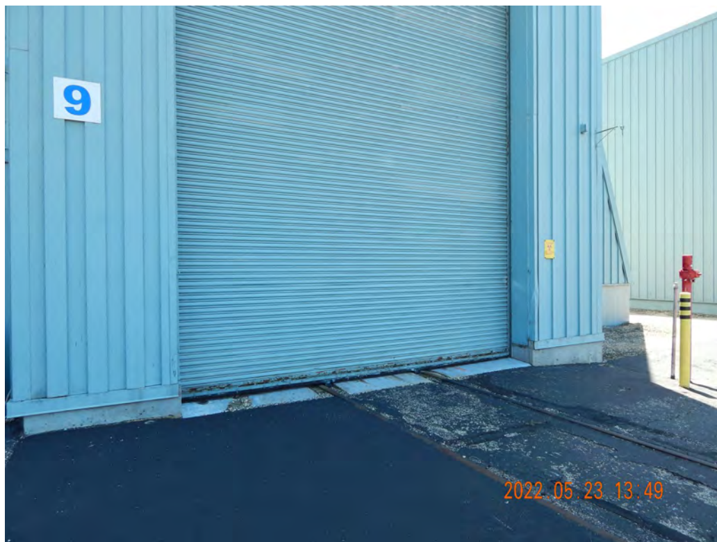
Figure 2-495. Railroad Tracks into the Cask Service Facility
