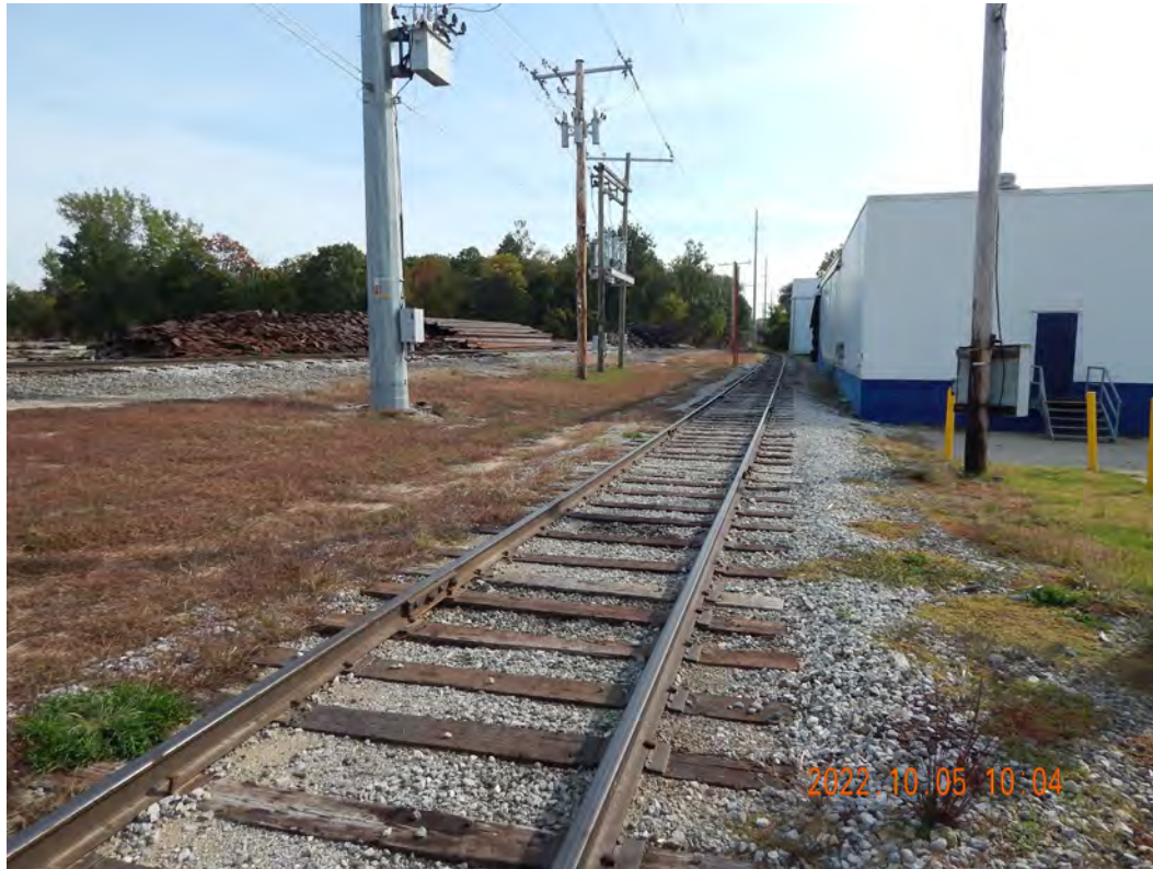
Figure 2-583. Lineage Logistics Potential Transload Location Looking East
