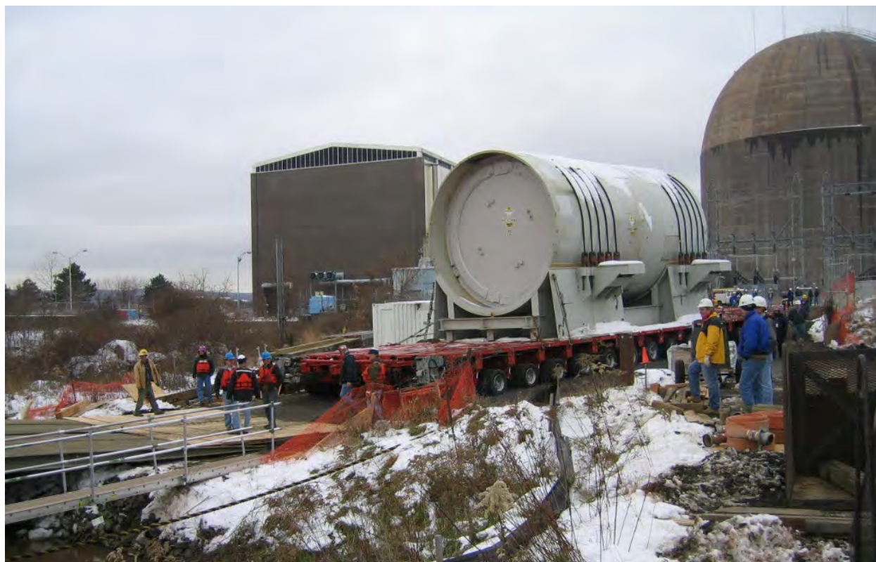
Figure 2-42. Connecticut Yankee Reactor Pressure Vessel Being Loaded onto Barge
