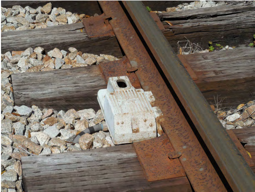
Figure 2-175. Hot Bearing Detector on Florida Northern Railroad (2015)
