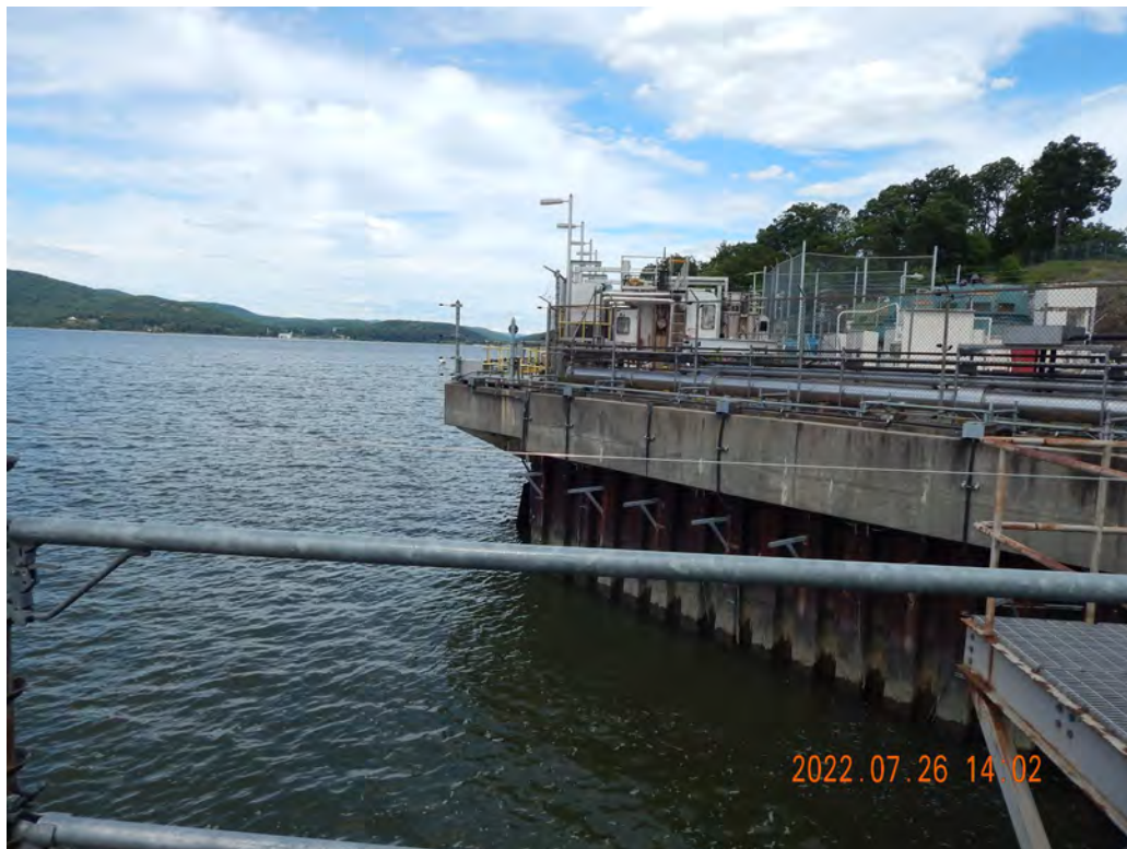
Figure 2-522. Indian Point Barge Area Looking North
