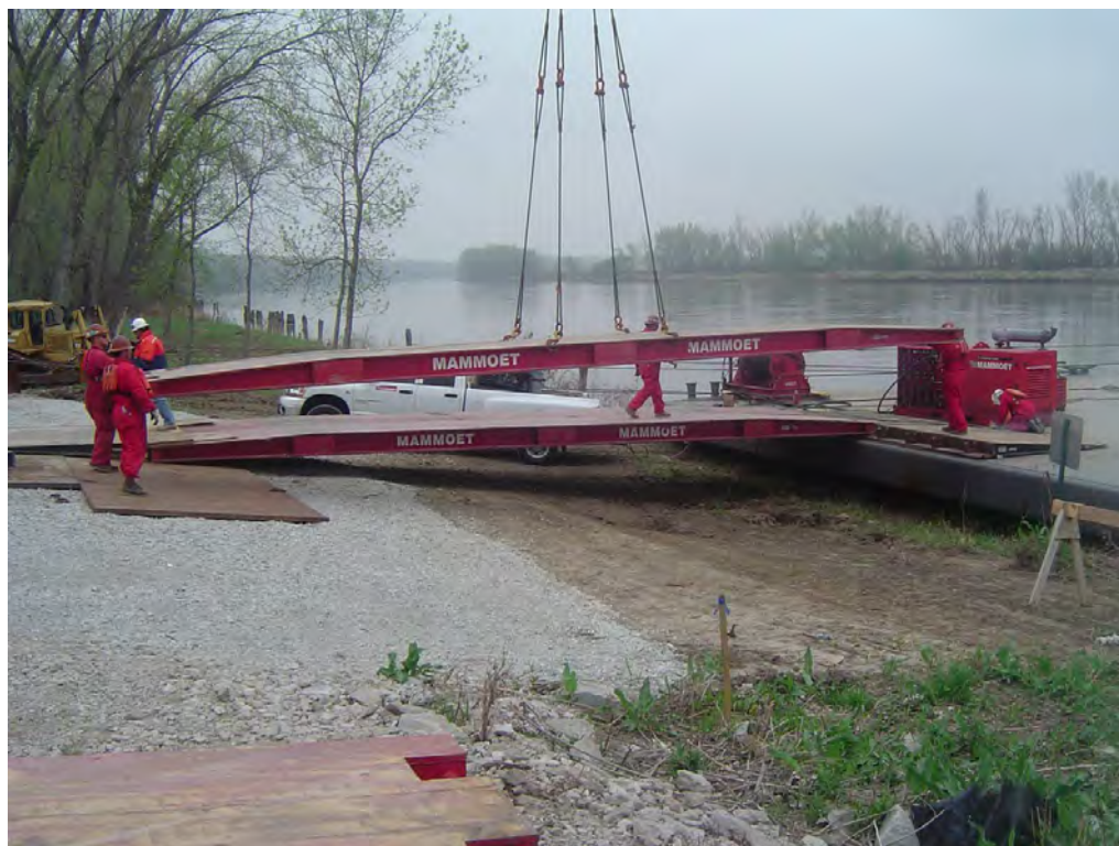
Figure 2-376. Installation of Temporary Ramps for Unloading (2006)
