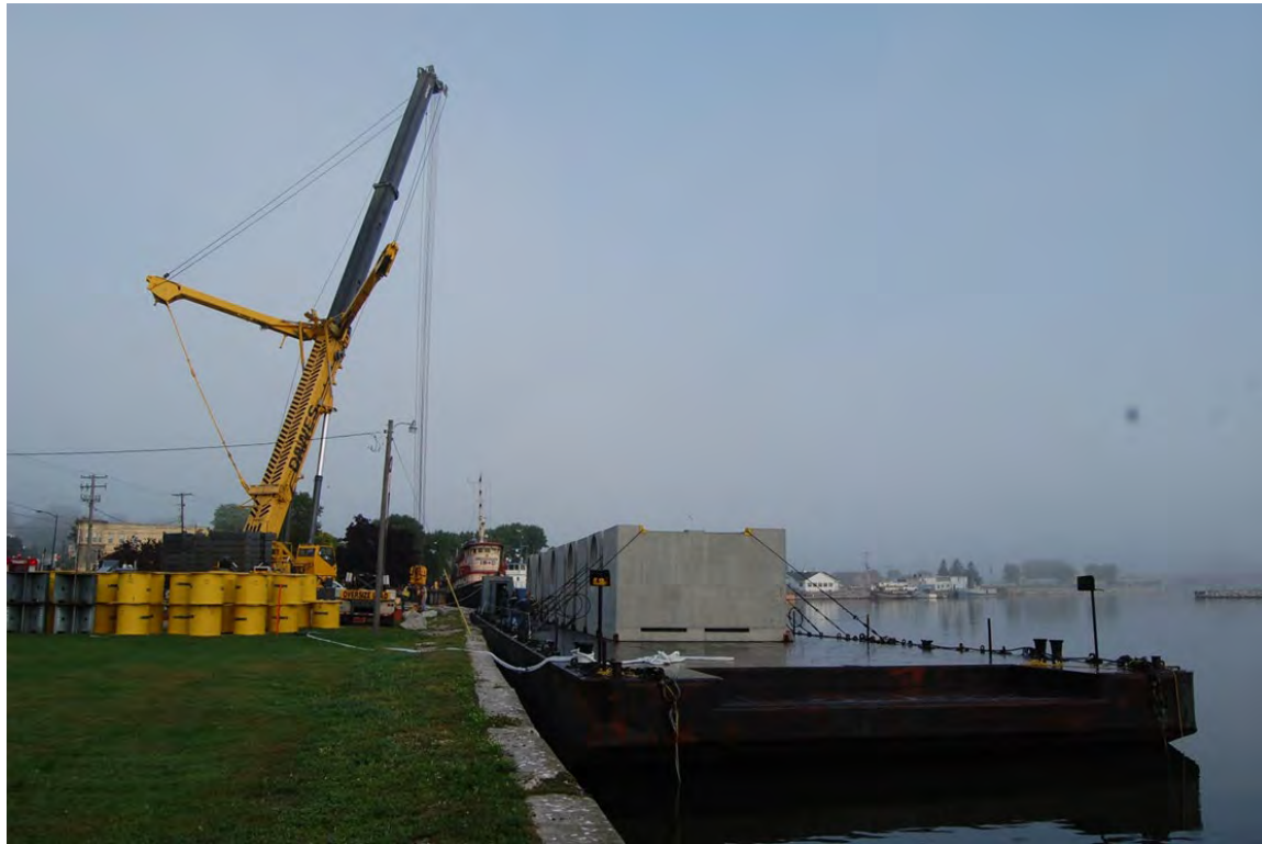
Figure 2-250. Horizontal Storage Modules Being Unloaded from a Barge (2013)
