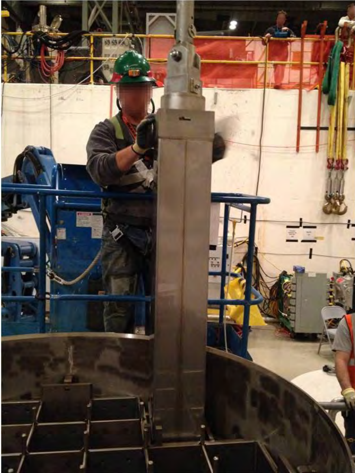
Figure 2-134. Damaged Fuel Can Being Installed in TSC-37 Canister
