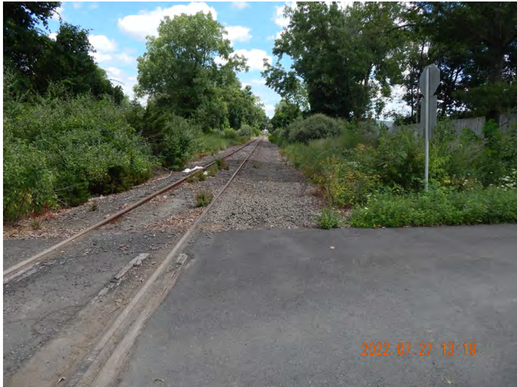
Figure 2-545. Agriventures Agway Potential Transload Location Looking Southeast
