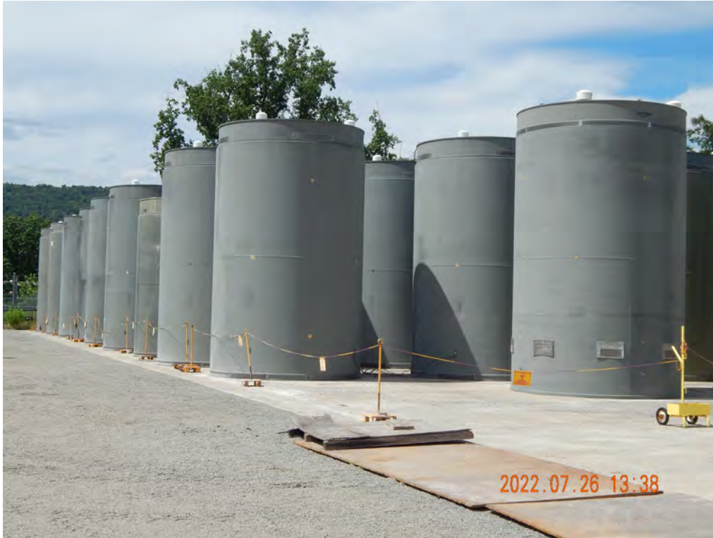
Figure 2-511. HI-STORM FW Dry Storage Systems at the Indian Point ISFSI (Looking West Towards Hudson River)
