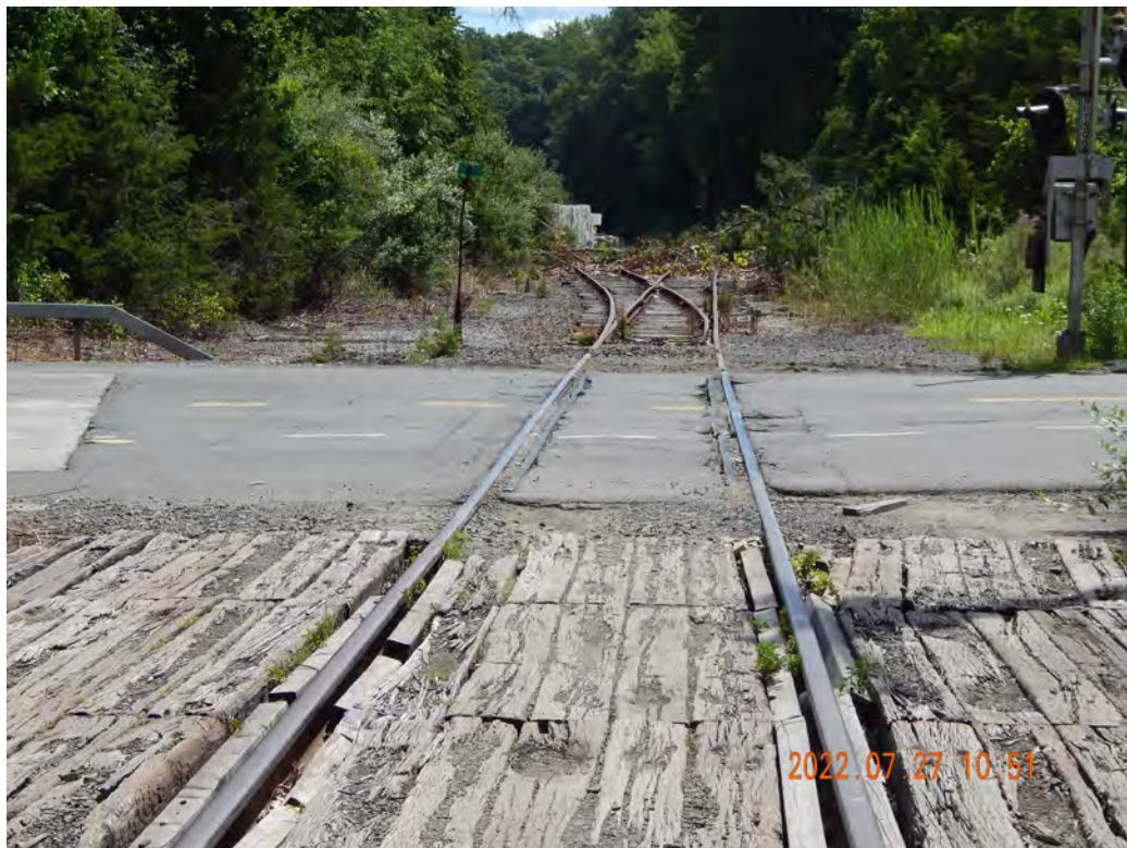
Figure 2-540. Segar Street Potential Transload Location Looking Southeast
