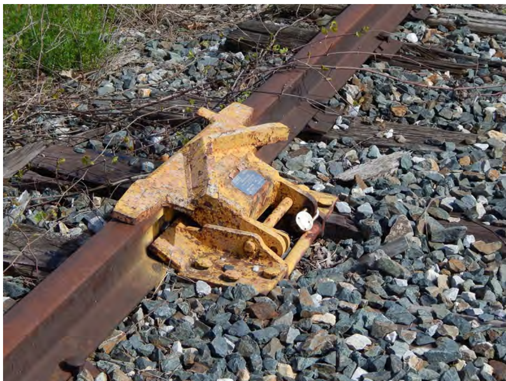
Figure 2-330. Derailer on Vermont Yankee Rail Spur (2016)
