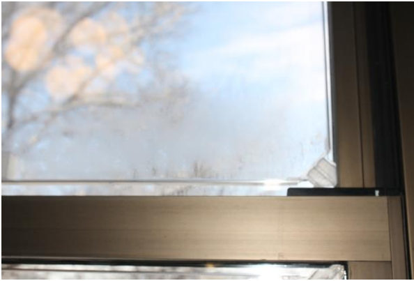
(c) Window attachments in the corners of the window lite hold the panel in place.
