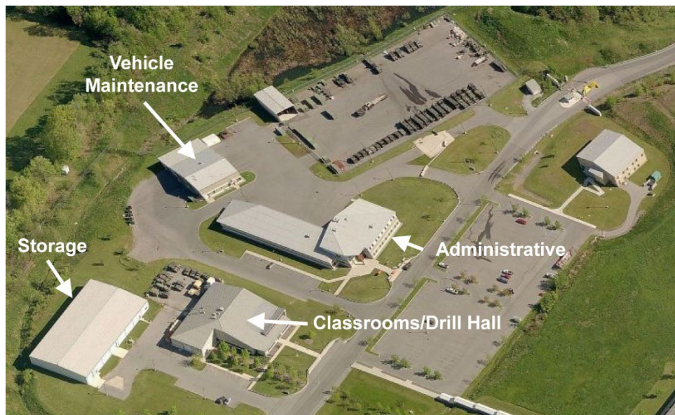
Figure 4. A Typical Army Reserve Center
