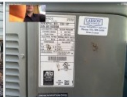
HVAC Unit 2 plate
