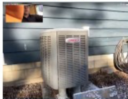
HVAC Unit 2 photo
