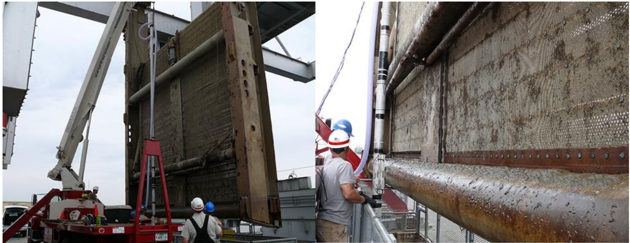
Figure A.18. For the baseline turbine characterization at Ice Harbor Dam stainless steel (SS) release pipes were attached to support frames of the submersible traveling screen in Slot B of Unit 1.
