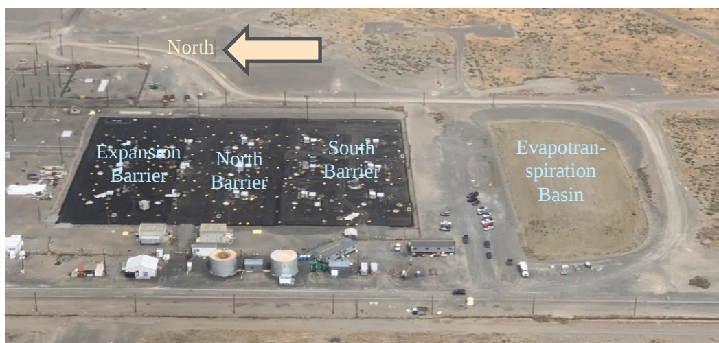
Figure 2. The SX tank farm with the interim surface barriers and the evapotranspiration basin.
