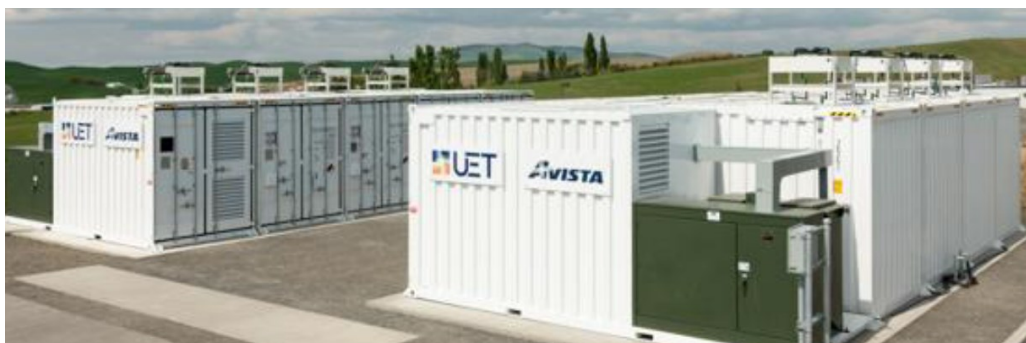
Figure 2.1. 1 MW, 3.2 MWh FBESS at Schweitzer Engineering Laboratory (SEL). Two strings each containing four battery modules and a Power Conversion System (PCS) container with Battery Management System (BMS) are shown.
