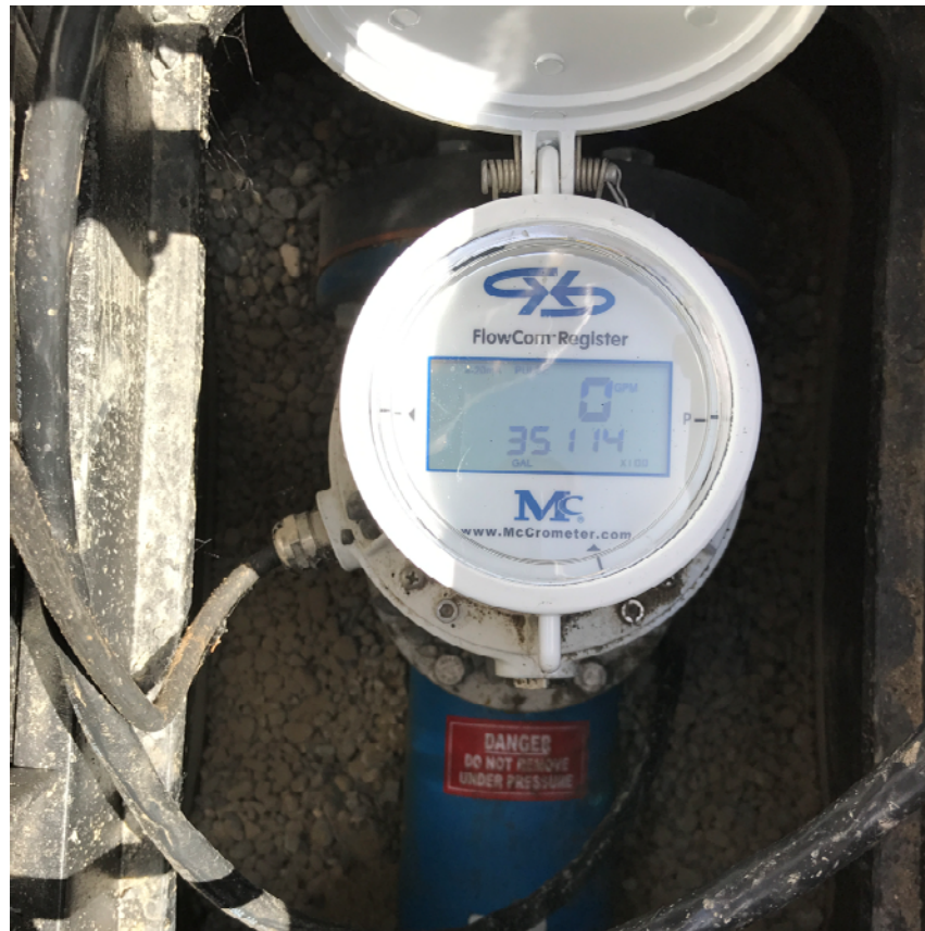
Figure 13. Irrigation Meter Installed at 3860 EAB
