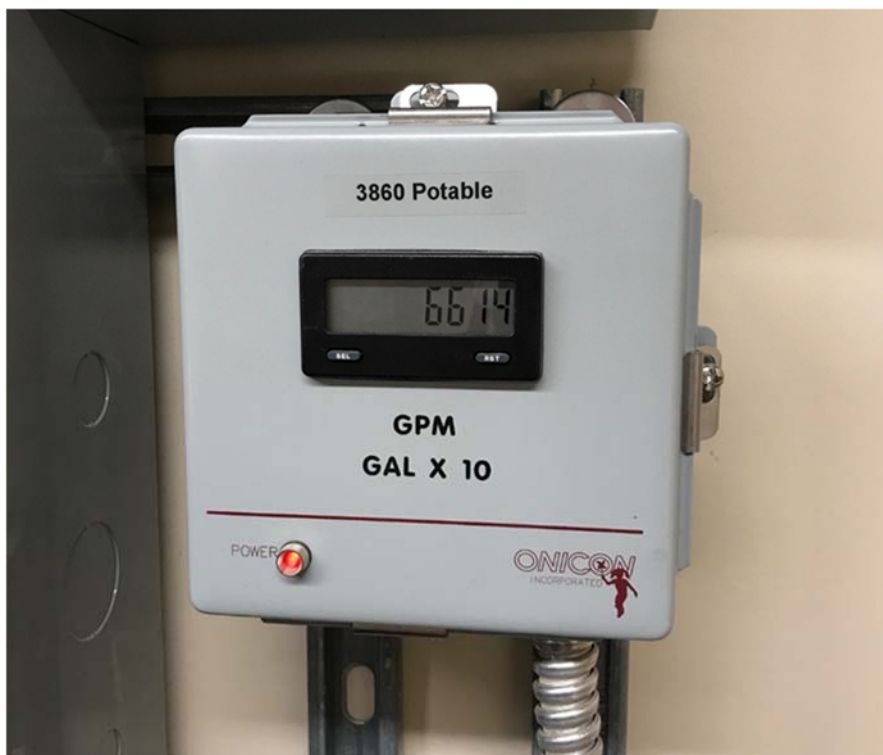
Figure 11. Onicon Water Meter Local Display in Room 123
