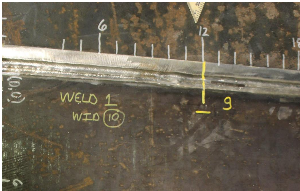
Figure 7.12. Photograph of Notch “g” Located in the Transition Weld
