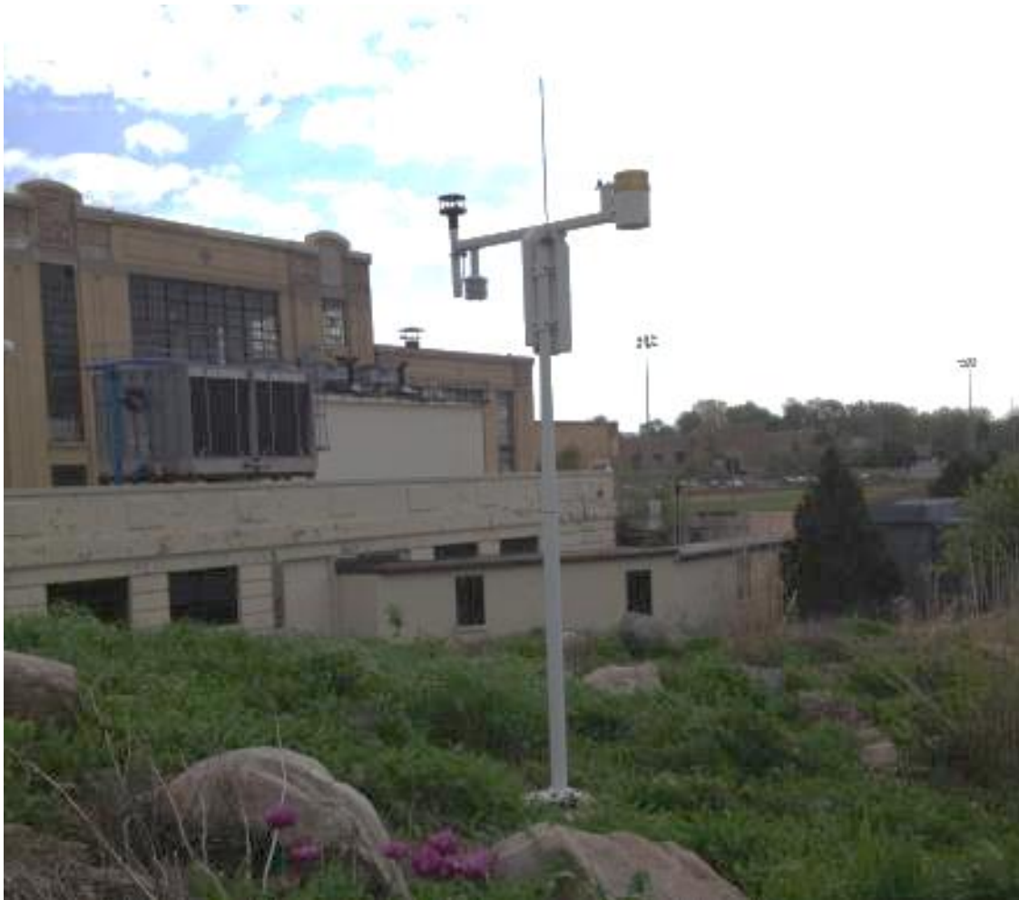
Figure 8. Weather Station at Hart-Dole-Inouye Federal Center
