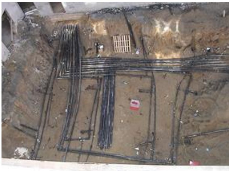
Figure 22: Piping for Ground Source Heat Pump Systems (DOE 2012b)
