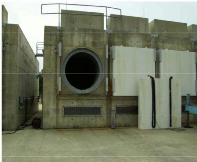
**Figure 1.2.** Typical NUHOMS Storage Module in Calvert Cliffs Nuclear Power Station ISFSI, Showing Front Air Inlet Vent and Open Doorway for DSC Insertion (from ISOE 2012)
