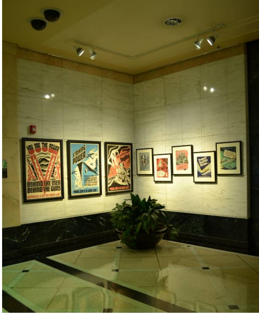
Figure 6. Lobby poster art lighted with Cree LRP38 LED lamps (AFTER). (Photo by Mike Hoffman, PNNL.)
