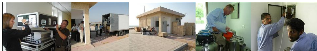
Figure 2.10. From Left to Right: Packing of the SAUNA in Stockholm, delivery at the station the boxes in front of the station, filling of the lead shields and making electrical connections.
