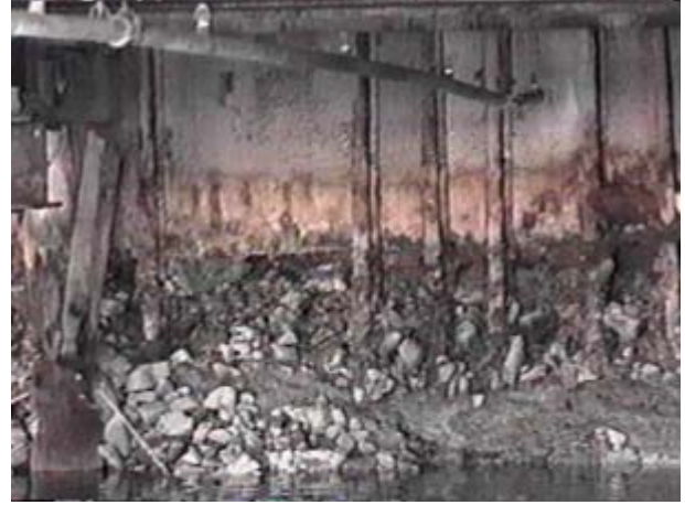
(b) Deteriorating bulkhead, approximately Transect +7.5
