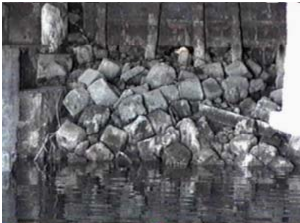
(e) Blocks of fill below vertical wall, approximately Transect +43.5
