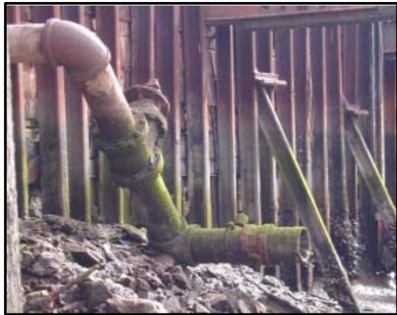
(c) Valved L-shaped pipe near Transect -24.5
