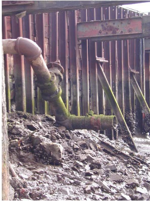
Photo 7 - 'L'-shaped pipe with gate valve. 2/6/02.
