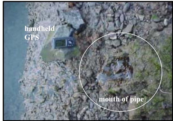
(d) Previously undocumented broken concrete pipe with water flowing, near Transect -8.5
