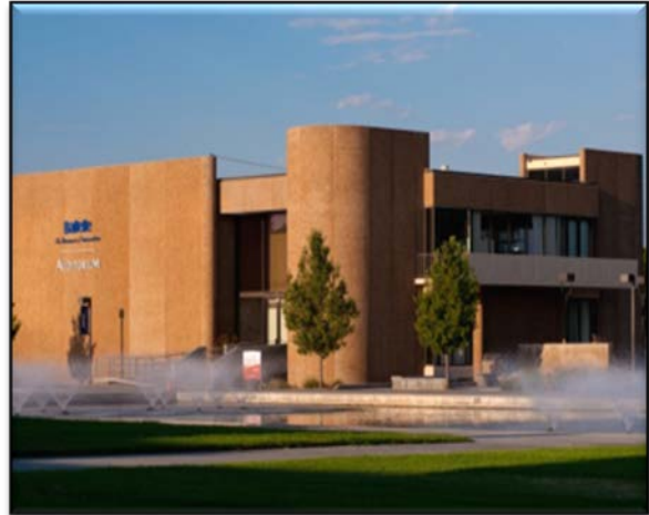
South campus Auditorium; open space central to staff core
